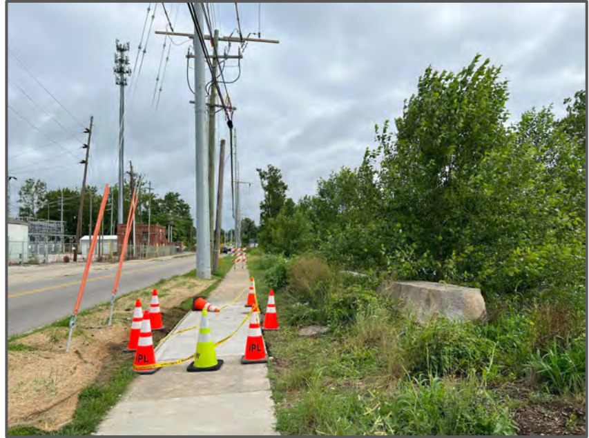
Replace Sidewalk Rogers Street
