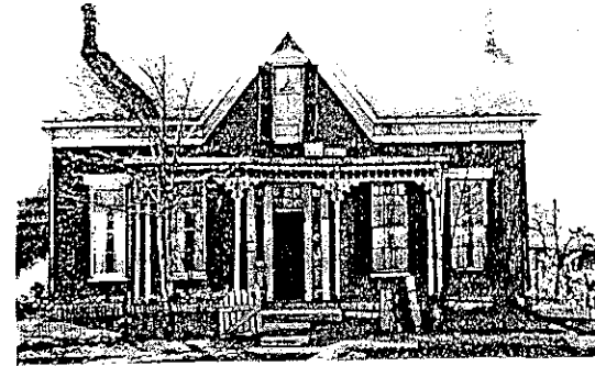
119 House. Photo courtesy Bloomington Restorations, Inc.
