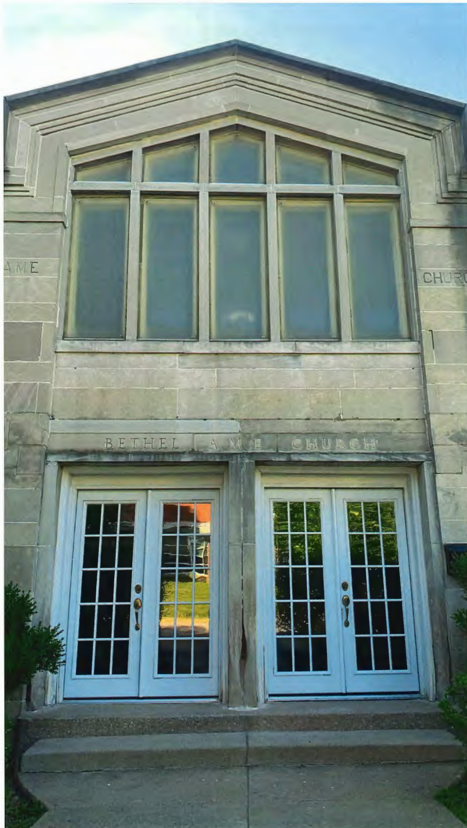
Image 8: Front of the church structure facing west, stone lintel with the A.M.E. carved, 2022 (photo by staff)
