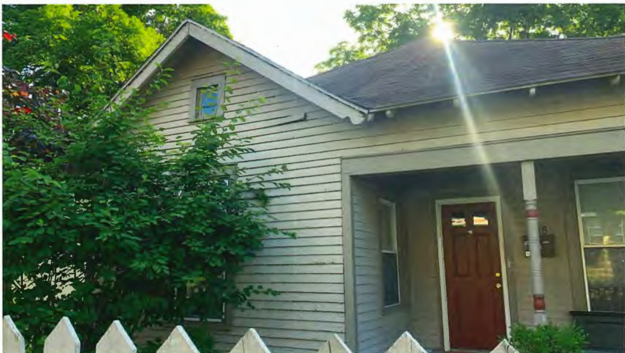
Image 12: West facade with the front entrance of the parsonage, bungalow, 2022 (photo by staff)
