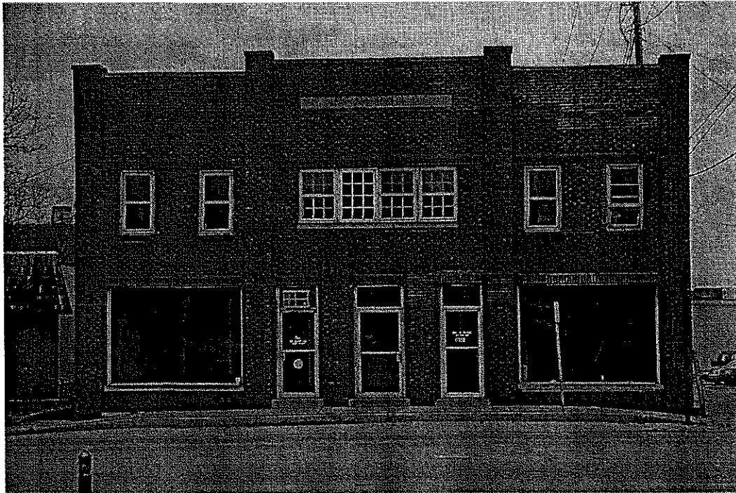
Fleener Building 112 East 3 rd Front Facade
