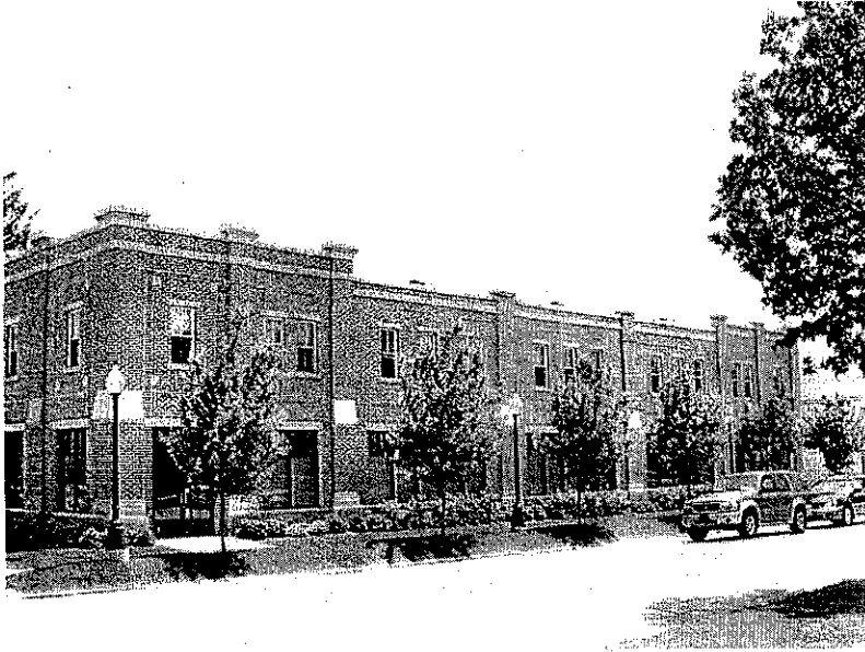
New construction: 6 th and Madison
