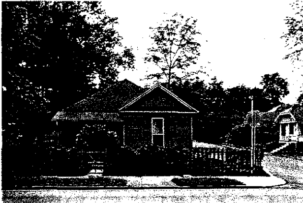
835 W KIRKWOOD - BLOOMINGTON RESTORATIONS, INC., HOUSE REHAB
