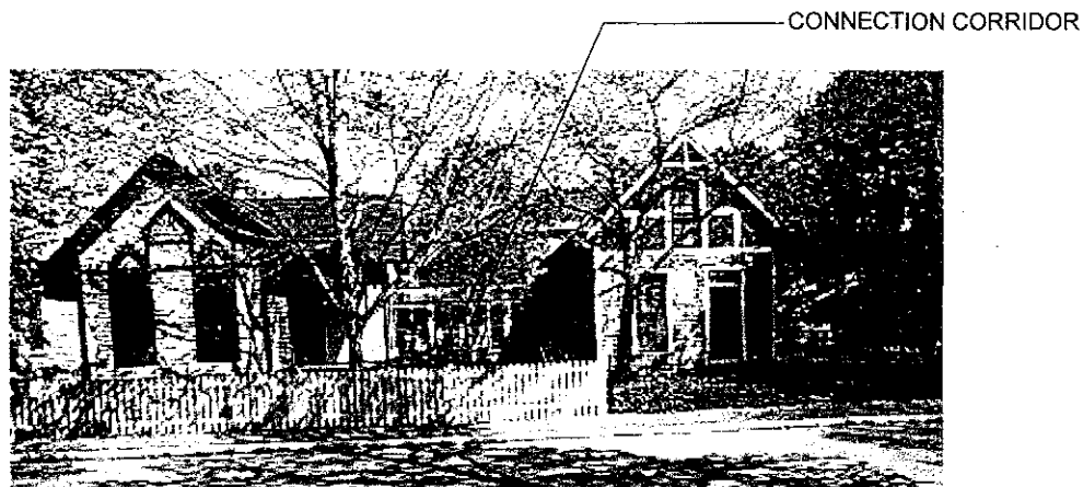
CONNECTED HOUSES IN LOCKERBIE, INDIANAPOLIS, CREATE LARGER SQUARE FOOTAGE WHILE RESPECTING SCALE OF NEIGHBORHOOD
