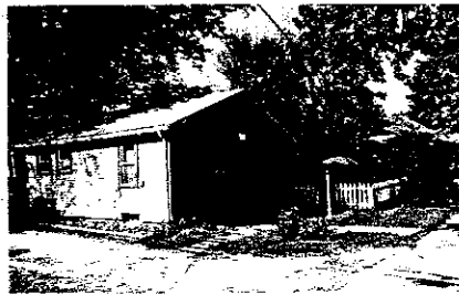
EXISTING ACCESSORY BUILDING OFF WEST KIRKWOOD
