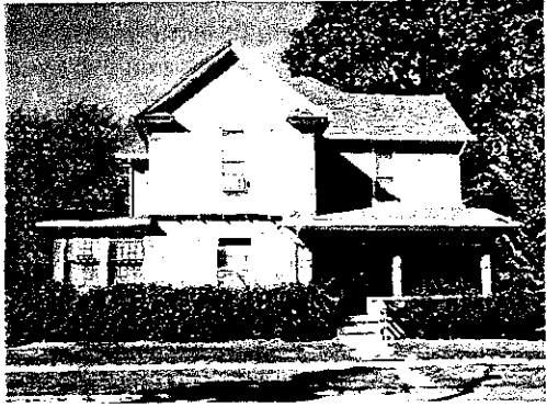
TWO STORY HOUSE ON WEST KIRKWOOD
