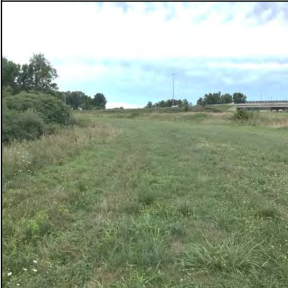
Photo 7: Grading on southern portion of Site; View to the south
