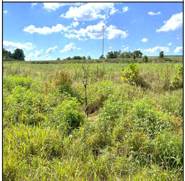
Photo 24: DP-8 excavation pit; View to the southeast
