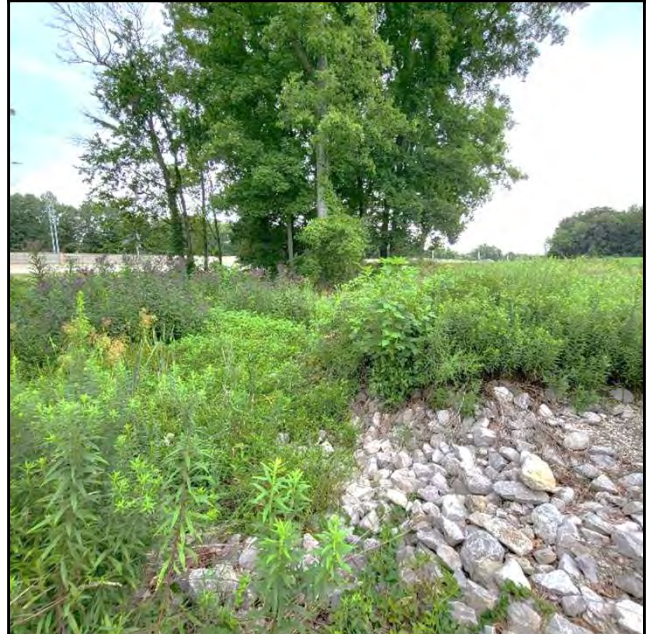
Photo 4: Rock check dam on the western Subject Property boundary; View to the northwest
