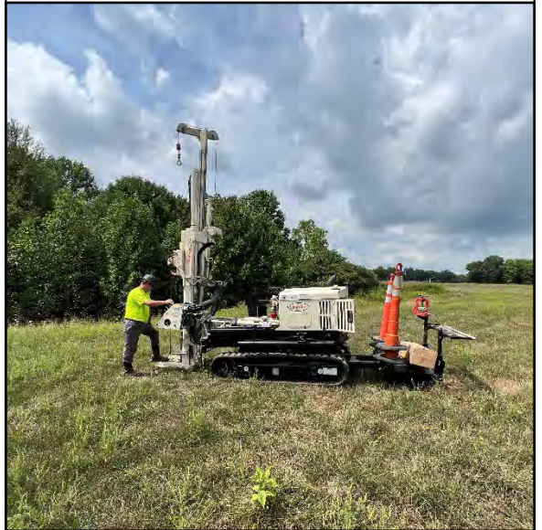
Photo 4: Drilling subcontractor advancing soil boring B-5; View to the west
