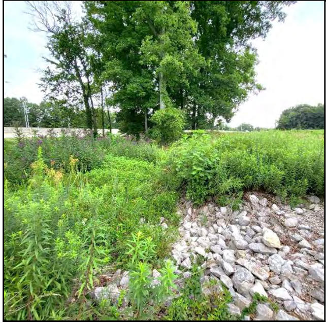
Photo 6: Rock check dam and Wetland #1; View to the northwest
