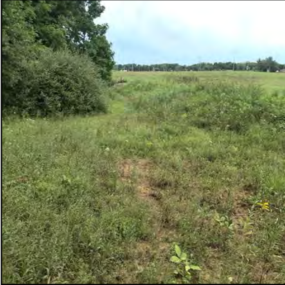
Photo 5: Northern terminus of man-made berm at northeastern Site boundary; View to the south
