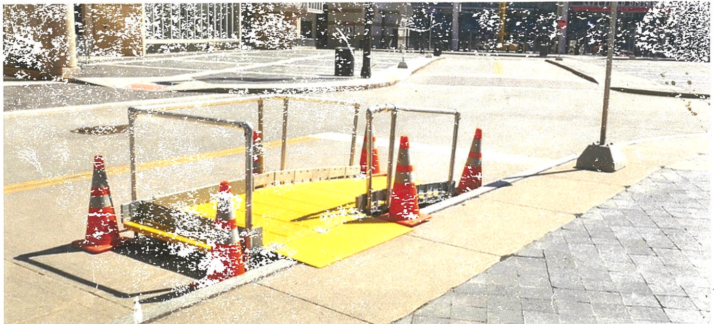
BoardWalk RAMP - Bi-Directional Platform 2 - Handrails - Right Turning from curb.
