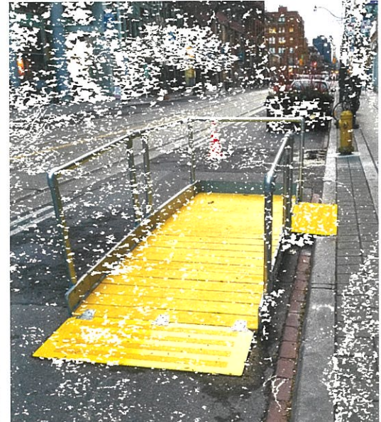
BoardWalk RAMP - Bi-Directional Platform 2 - Handrails - Left Turning from curb.
