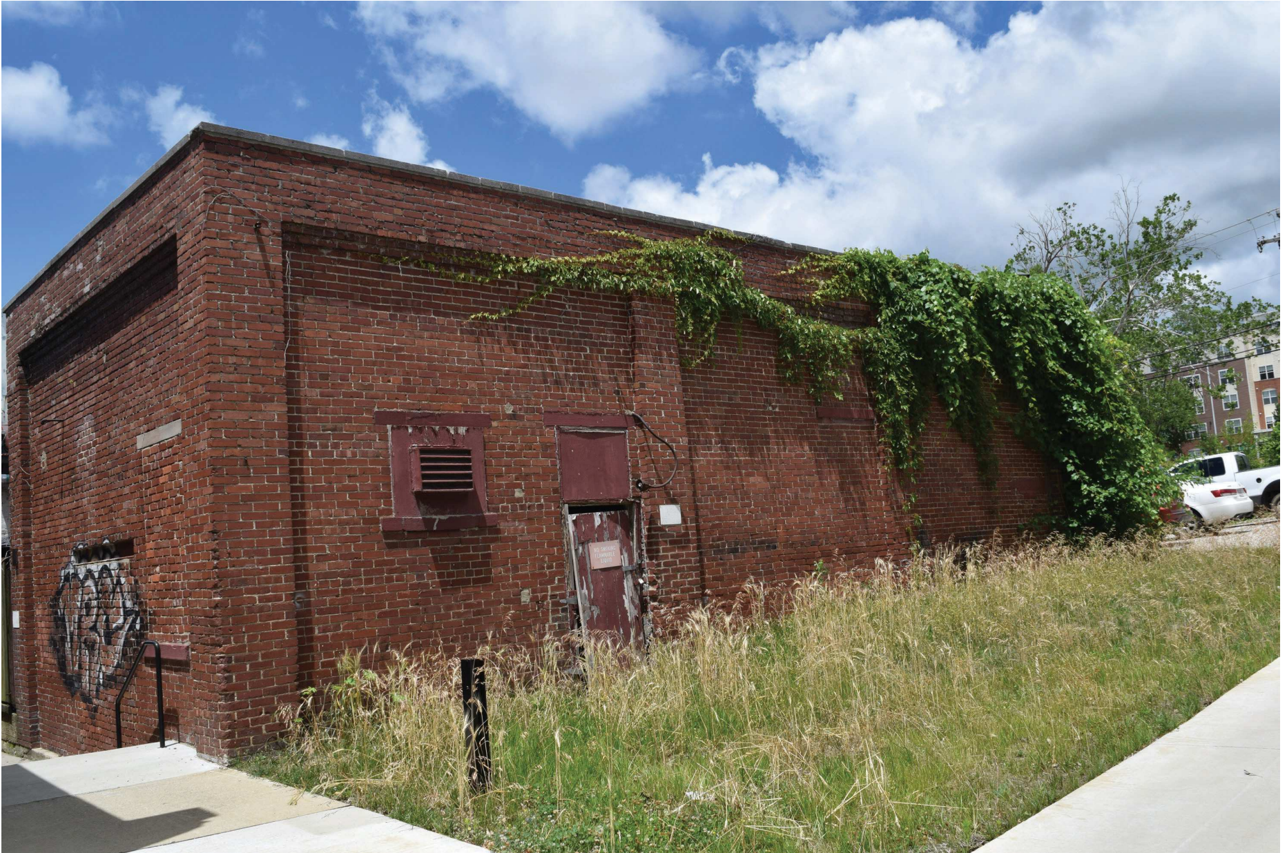
EXISTING POWER HOUSE STRUCTURE
