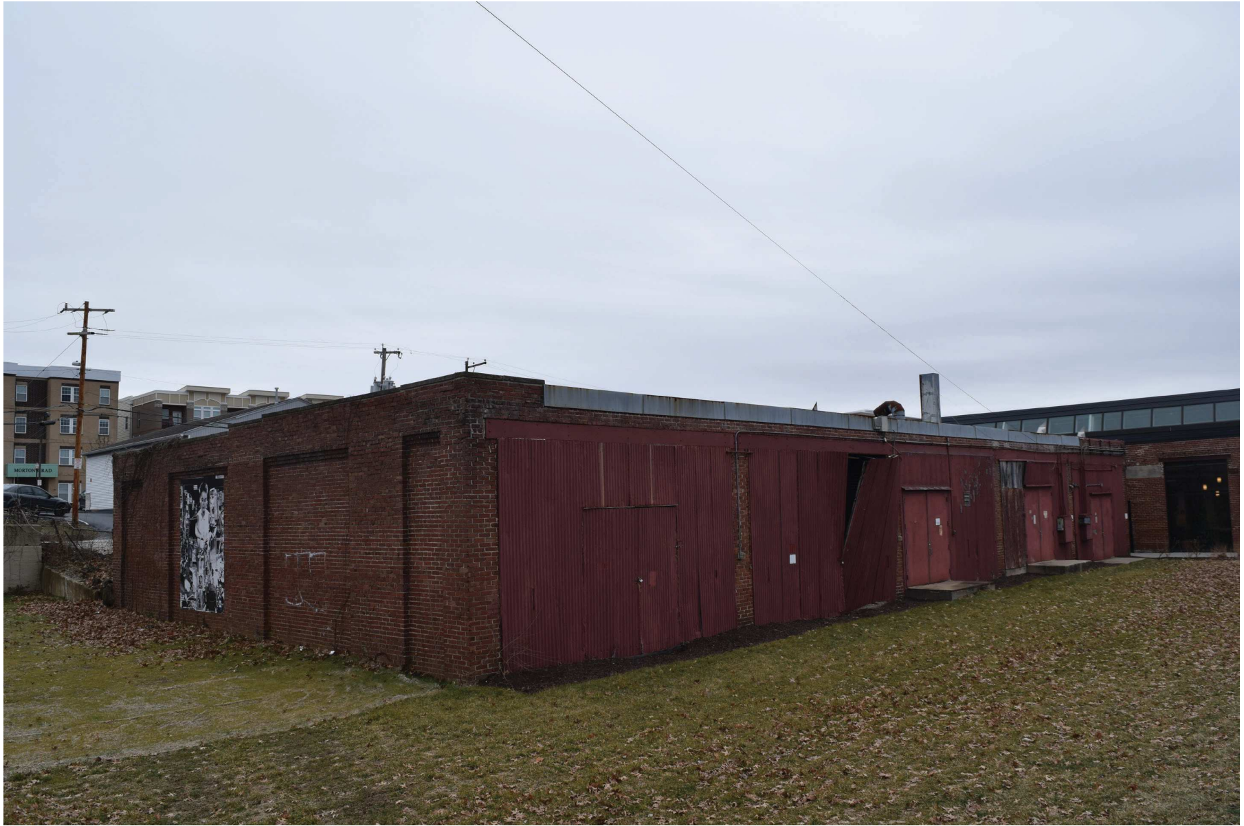
EXISTING KILN STRUCTURE
