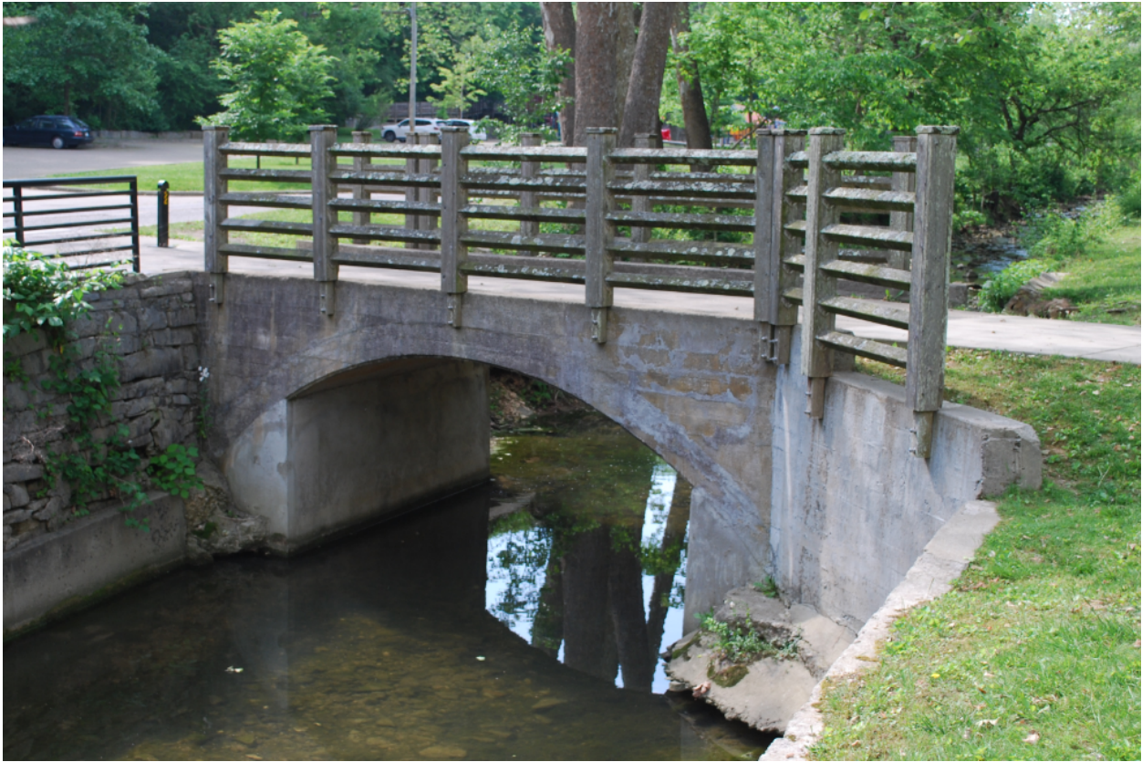
Image 7: Concrete Pedestrian Bridge, looking southwest
