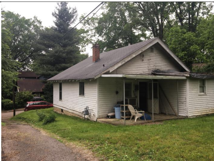
South Elevation, looking west along alley
