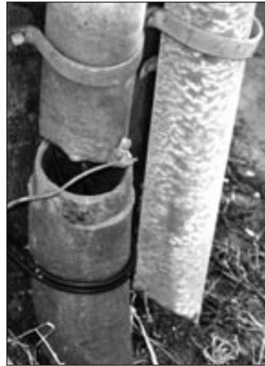
Steel U-Guard requires grounding strapping and does not have belled ends.
