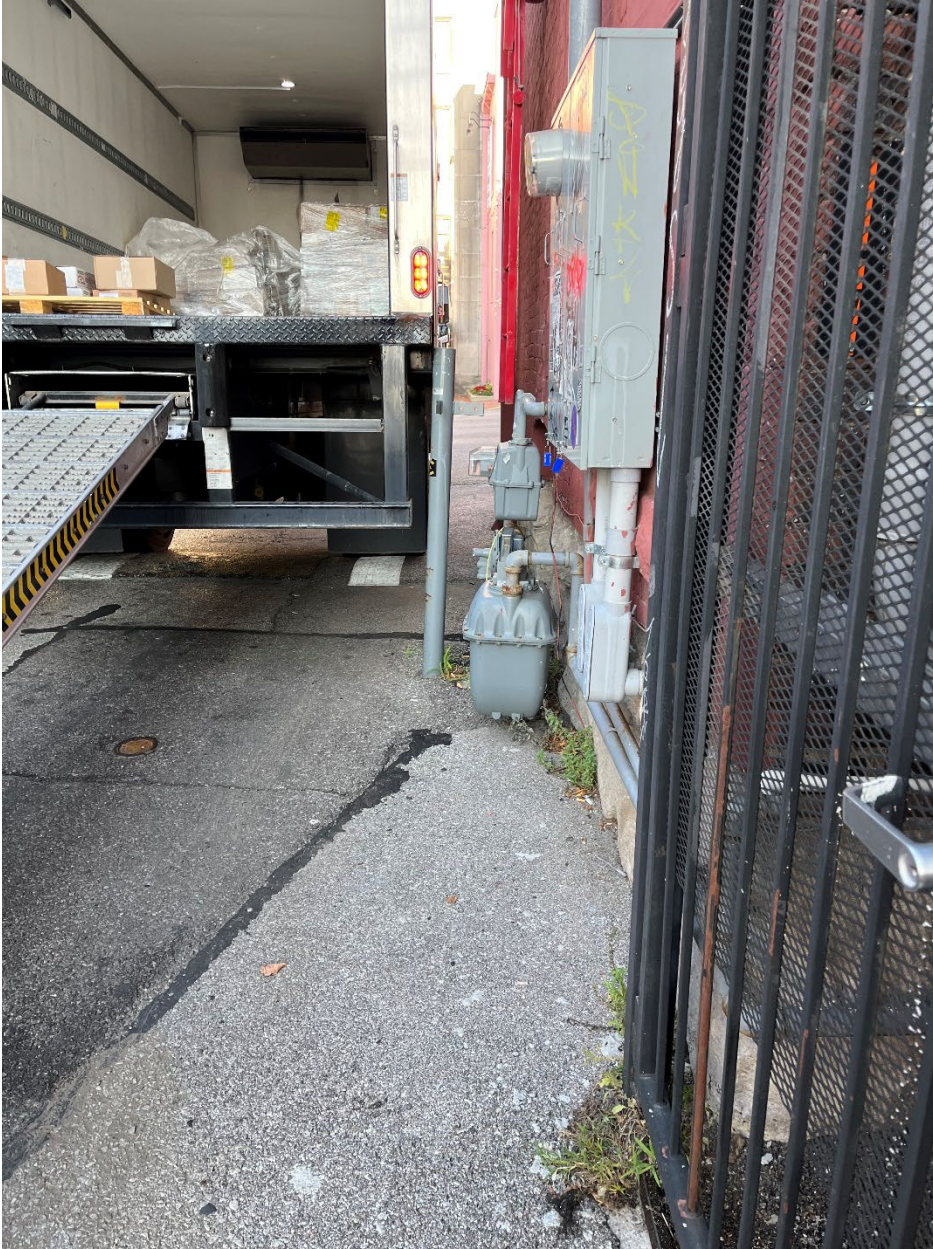
Alley looking west toward S. Walnut St. delivery vehicle parking in the alleyway. (1/2)
