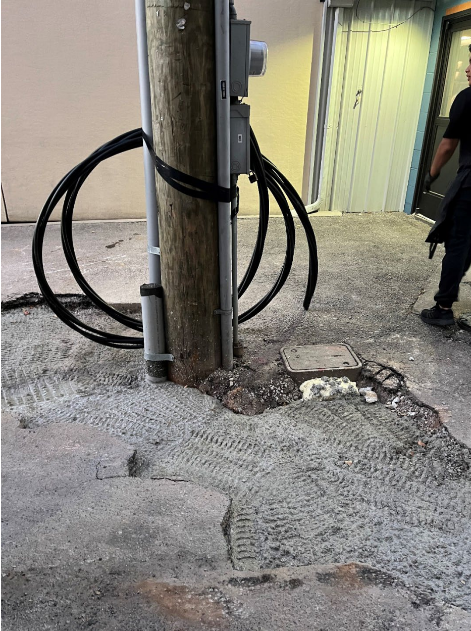
Newly installed Duke power lines from 8/31/23
