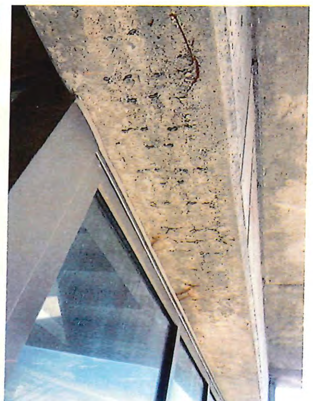
4 - beam cracks.JPG
