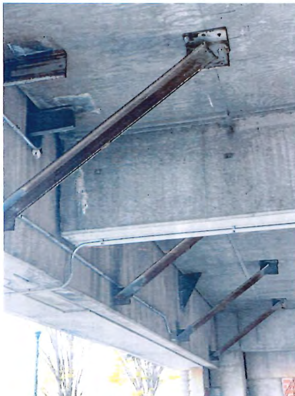
23 - corroded wall panel connection.JPG
