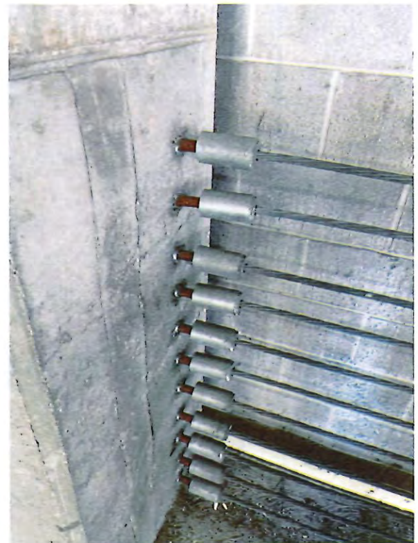
16 - corroded vehicular barrier cabling connection.JPG
