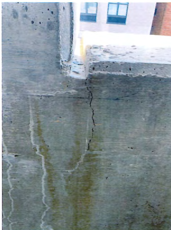
7 - exterior wall cracks.JPG
