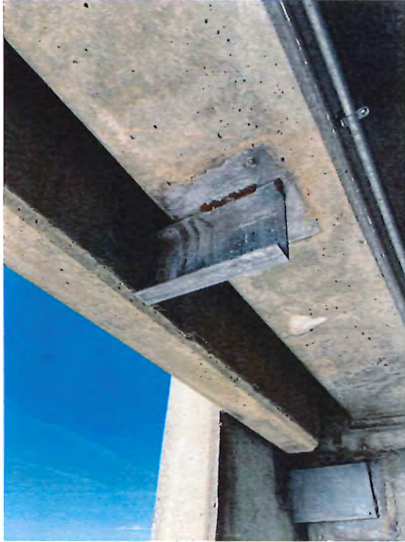
21 - corroded wall panel connection.JPG
