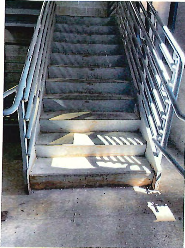
17 - stair steel corrosion.JPG
