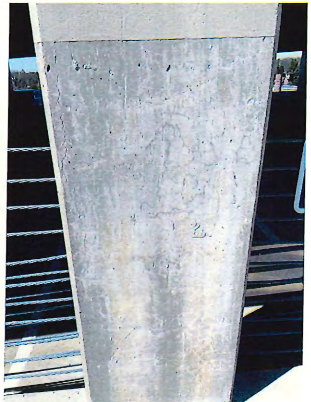
4 - column cracks with delamination.JPG
