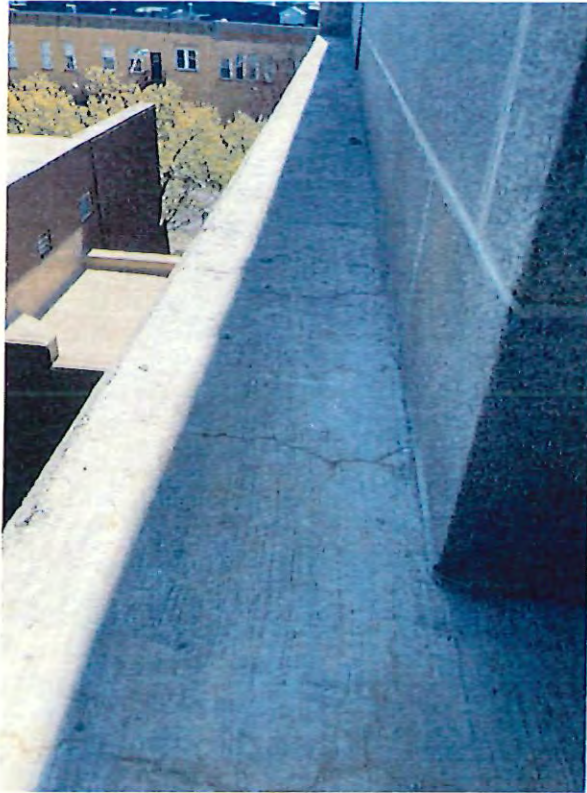
9 - exterior wall cracks.JPG
