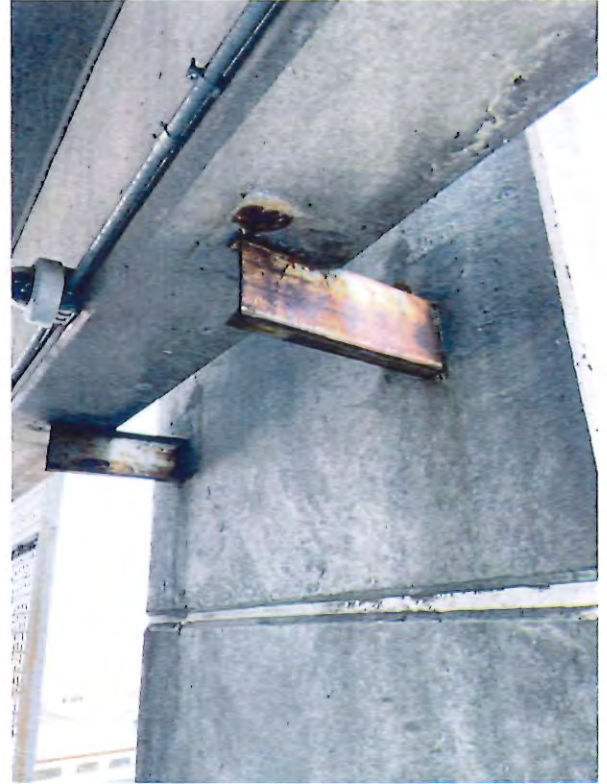
22 - corroded wall panel connection.JPG
