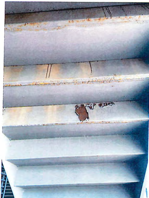
19 - stair steel corrosion.JPG
