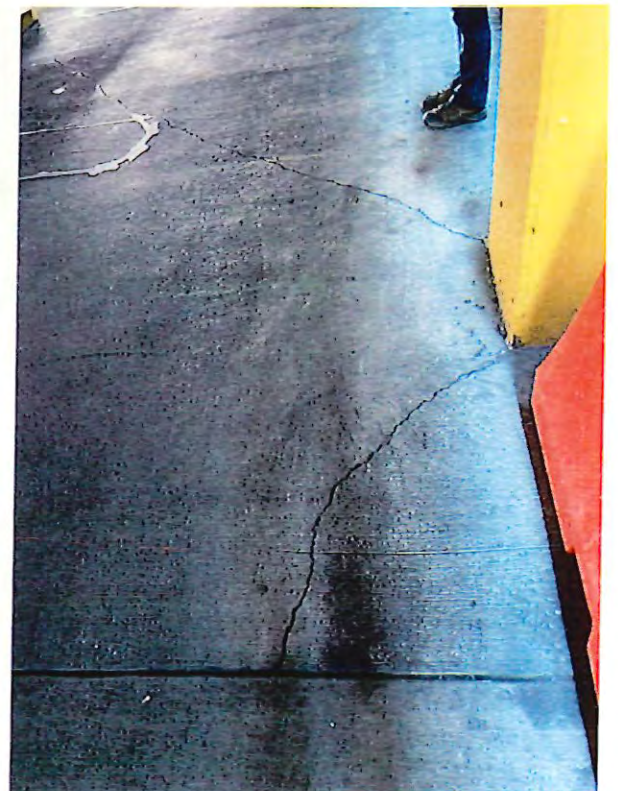
12 - SOG parking deck cracks.JPG
