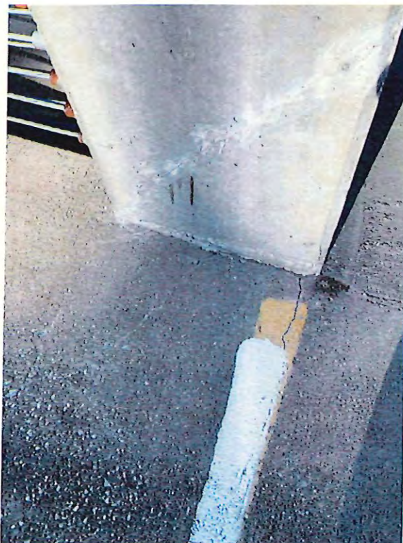
11 - elevated parking deck crack.JPG
