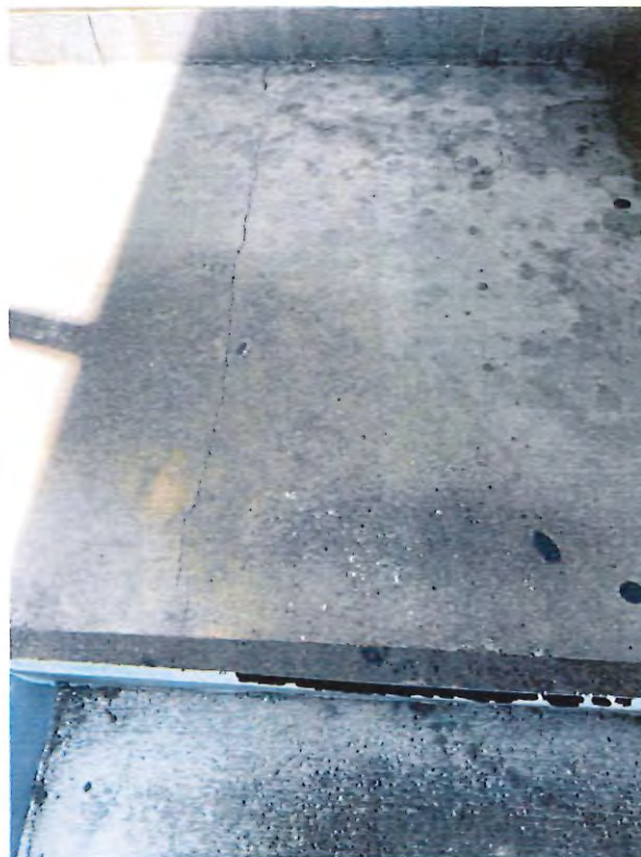
15 - crack in stair landing.JPG
