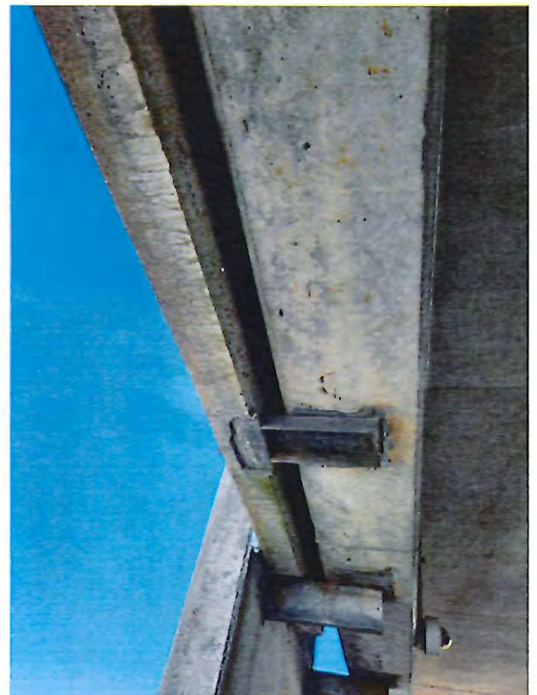
16 - spalled concrete at embed.JPG
