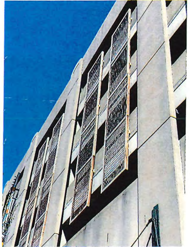
34 - facade panel corrosion.JPG
