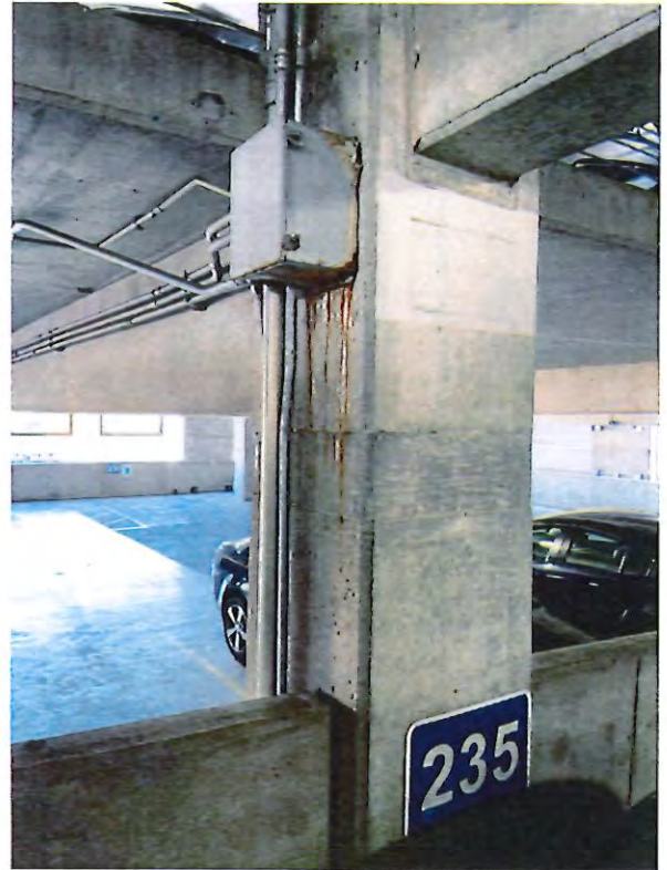
30 - corroded electrical box.JPG
