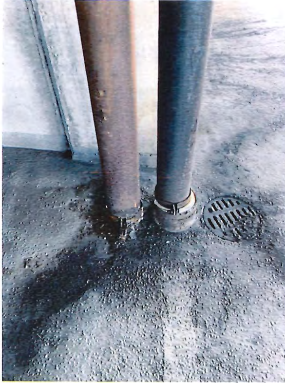
29 - corroded drain pipe and sleeves.JPG
