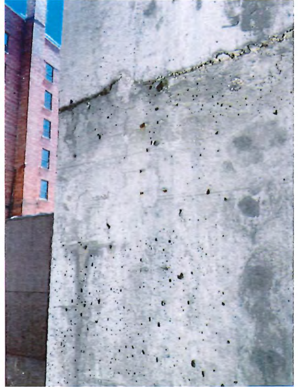
6 - column cracks with delamination.JPG
