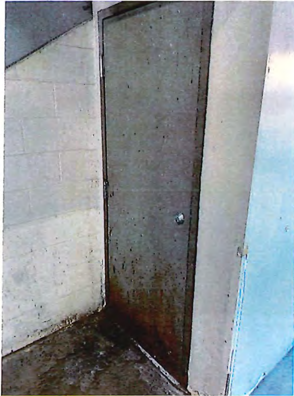
33 - door and frame corrosion.JPG
