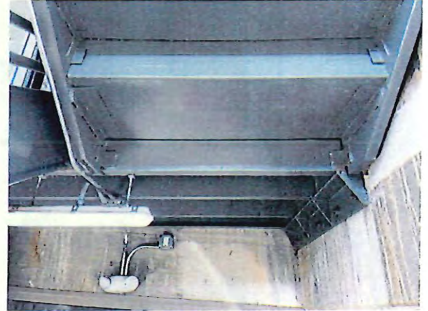
26 - east stair steel corrosion.JPG
