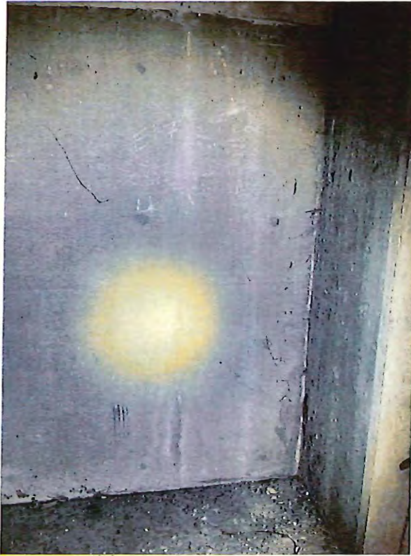
9 - basement level - wall crack.JPG
