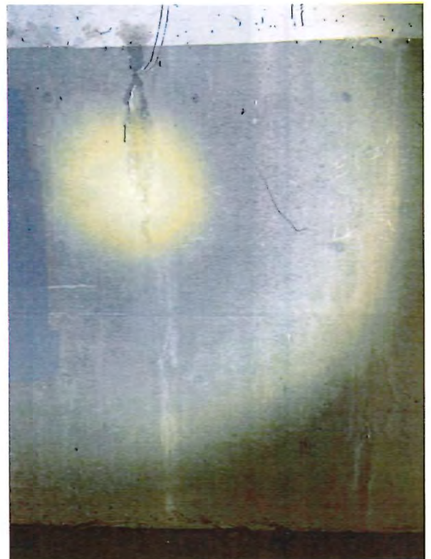
8 - basement level - wall crack.JPG
