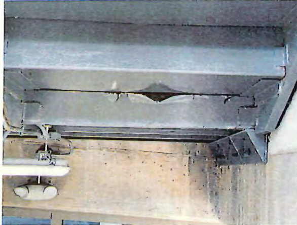
25 - east stair paint peeling and steel corrosion.JPG
