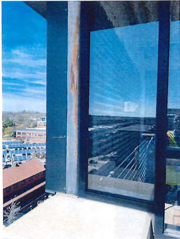
21 - stair tower steel corrosion.JPG
