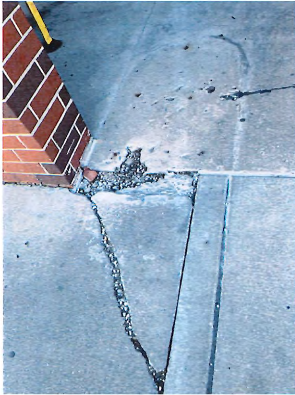
13 - SOG spalled concrete.JPG
