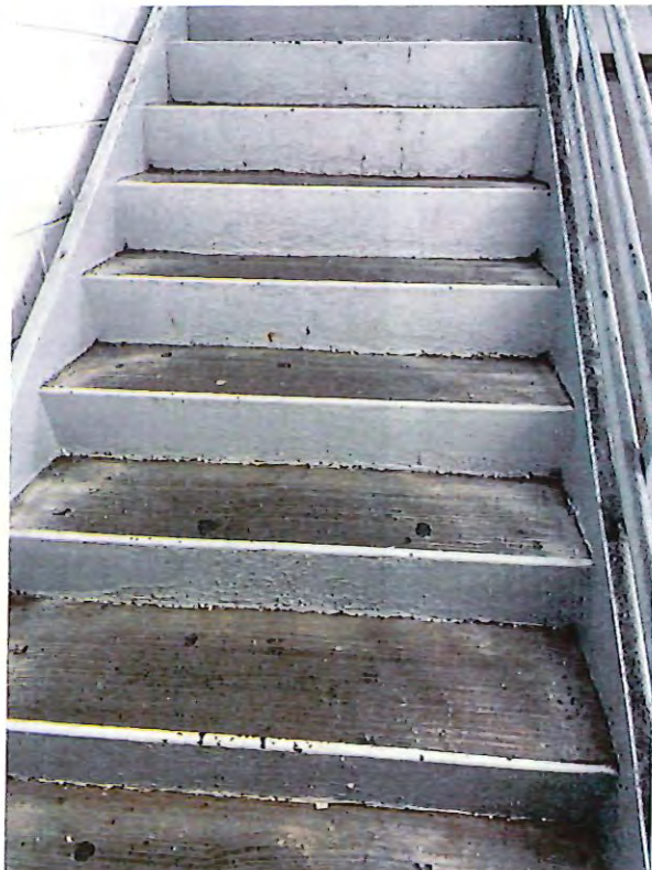
27 - west stair steel corrosion.JPG
