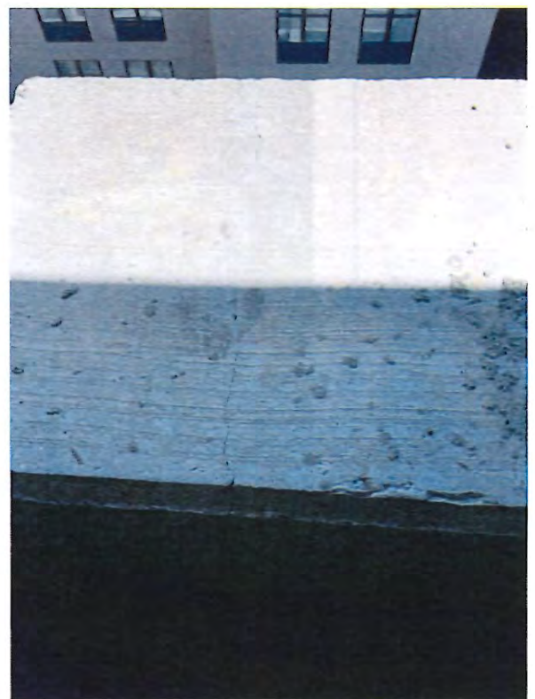
8 - exterior wall cracks.JPG
