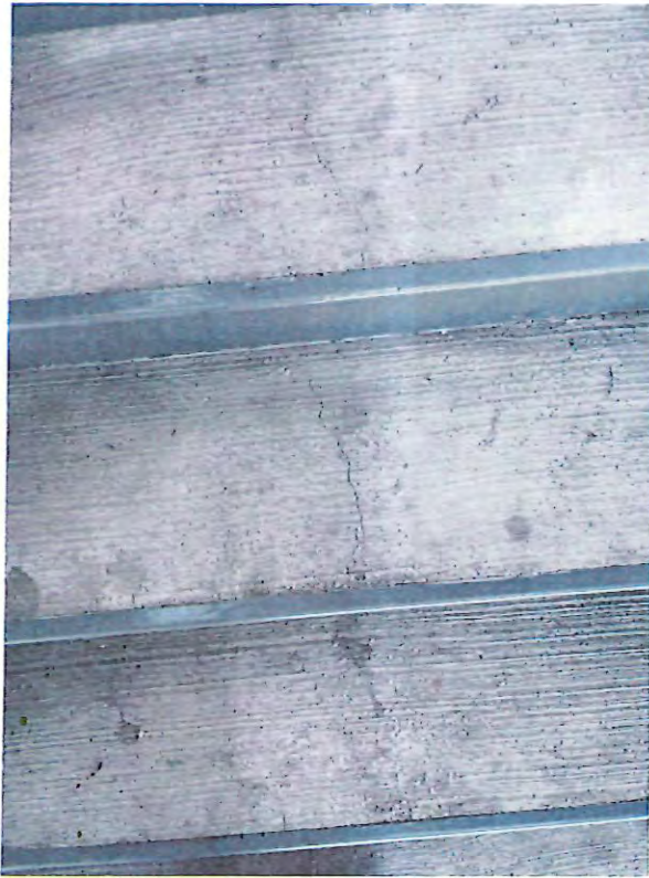
17 - crack in stair tread.JPG
