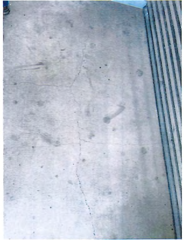
14 - crack in stair landing.JPG
