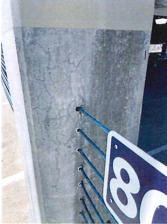
5 - column cracks with delamination.JPG
