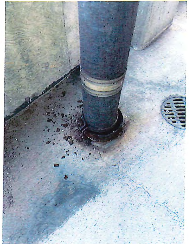
28 - corroded drain pipe sleeve.JPG
