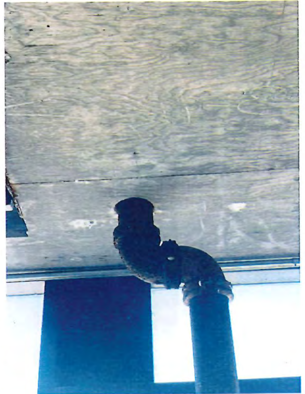
22 - pipe corrosion.JPG
