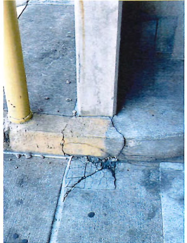
14 - spalled concrete curb.JPG
