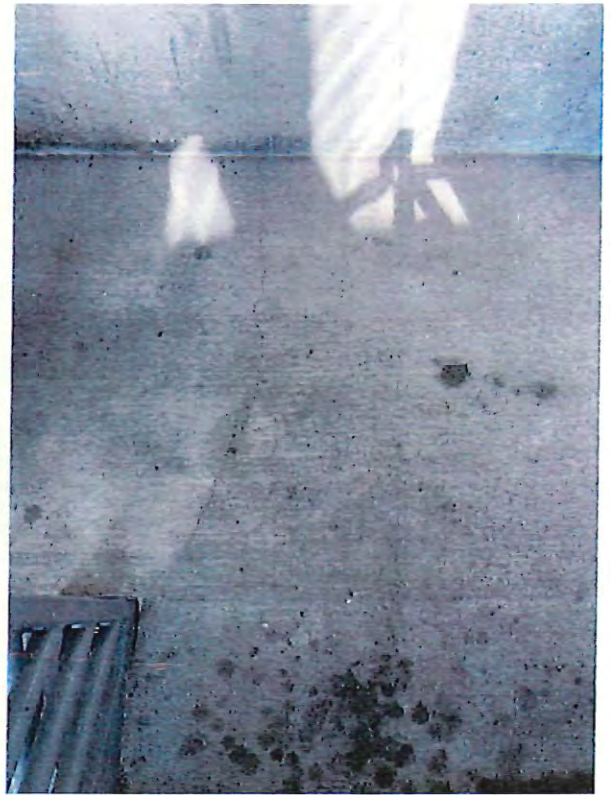
18 - crack in stair landing.JPG
