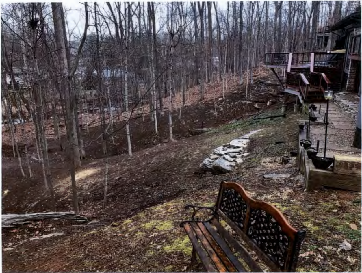
Photo 1: Disturbed land, including trees removed on steep slopes at 2408 S Shadow Grove Ct on 02/22/2024.
