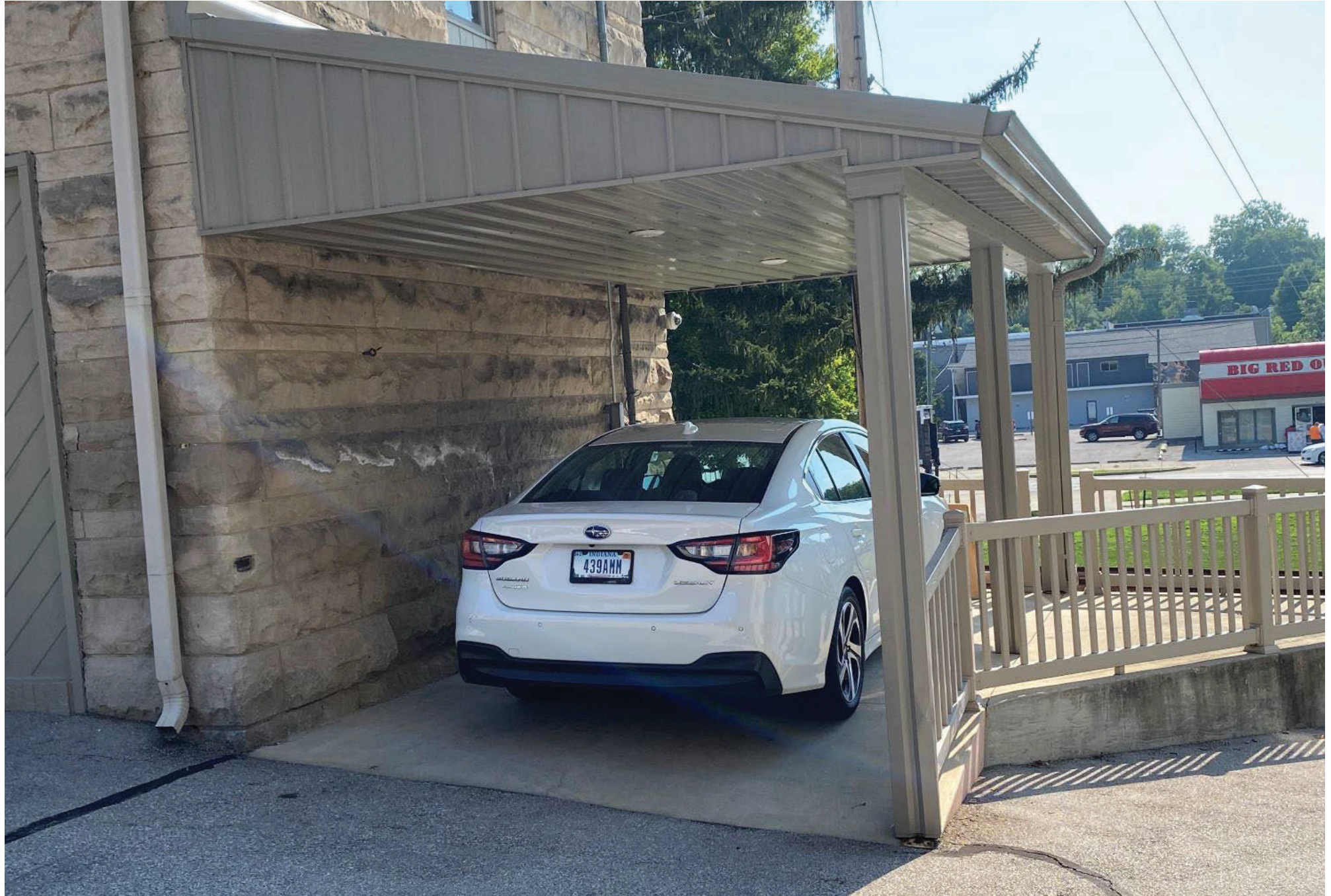
Carport on the side of the Red Cross building at College and 2 nd St.
