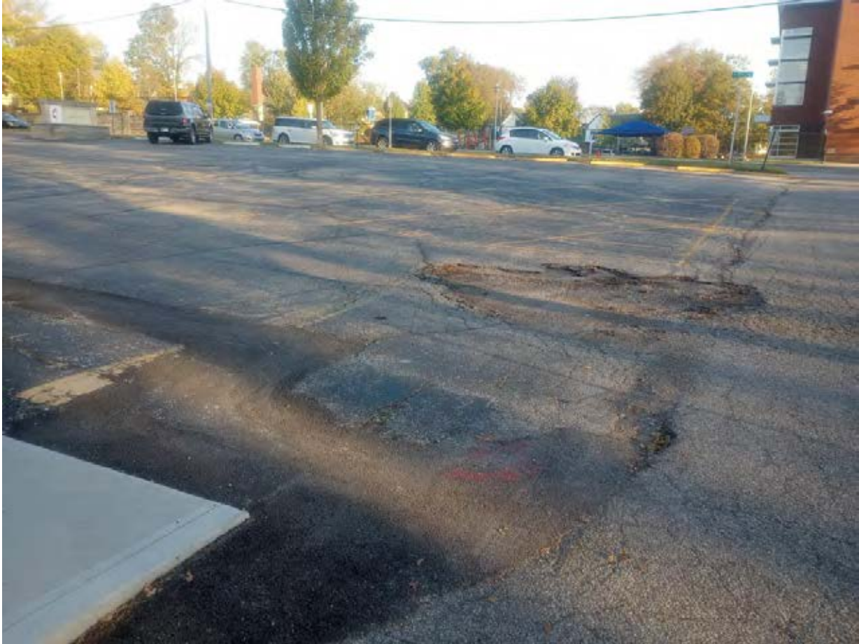
Existing partial pedestrian route on the west side of Jackson Street from 6th Street to 7th Street, edge of the church parking lot (looking south to north) 10/11/2024
