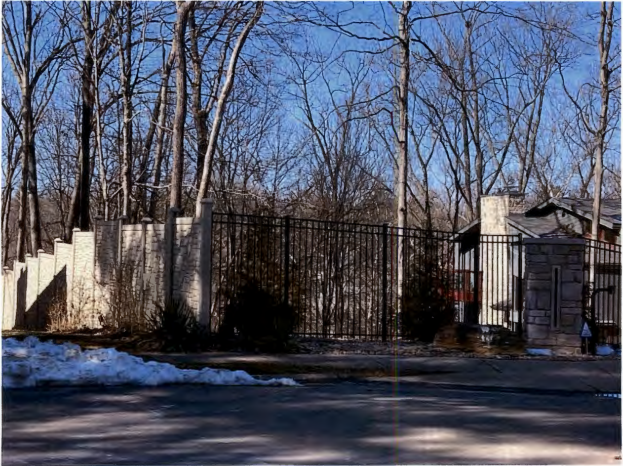
Photo 12: Fencing exceeding 4 feet forward of the front building wall at 2408 S Shadow Grove Ct on 02/20/2024.
