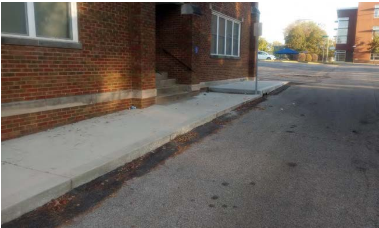
Existing partial pedestrian route on the west side of Jackson Street from 6th Street to 7th Street, third vertical step (looking south to north) 10/11/2024
