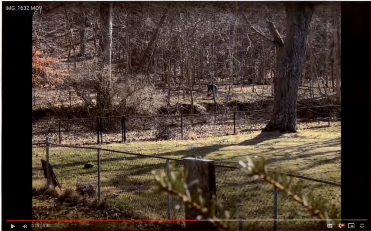
Photo 18: Screenshot of a video of a chainsaw being used to remove and chop up vegetation in the floodplain and riparian buffer on City-owned property adjacent to 2408 S Shadow Grove Ct on 02/29/2024 after the Stop Work Order (SWO) was issued on 02/22/2024.
