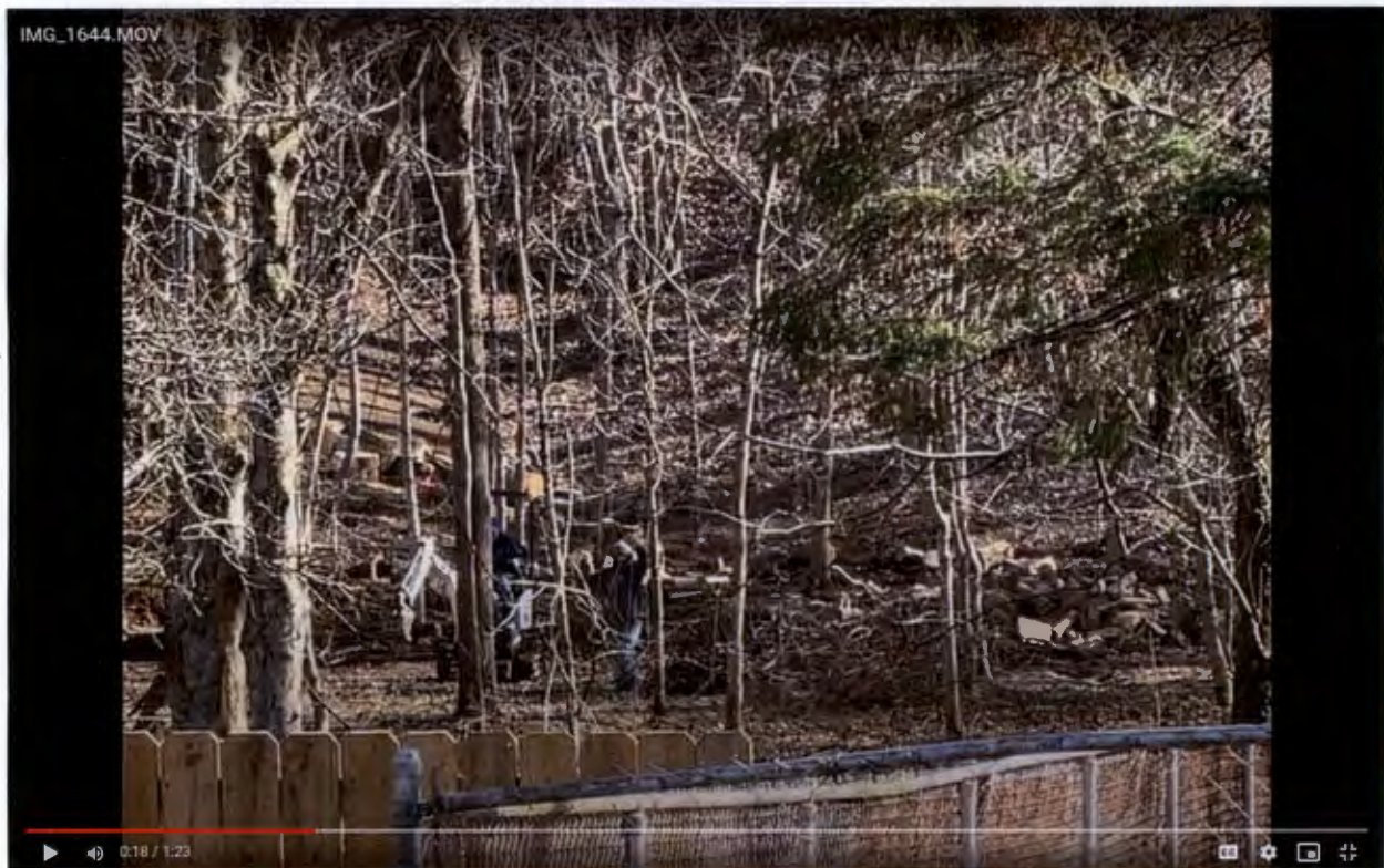
Photo 19: Screenshot of a video of the excavator operating on the property and being used to bring down vines on trees in the floodplain and riparian buffer on City-owned property adjacent to 2408 S Shadow Grove Ct on 02/29/2024 after the Stop Work Order (SWO) was issued on 02/22/2024.
