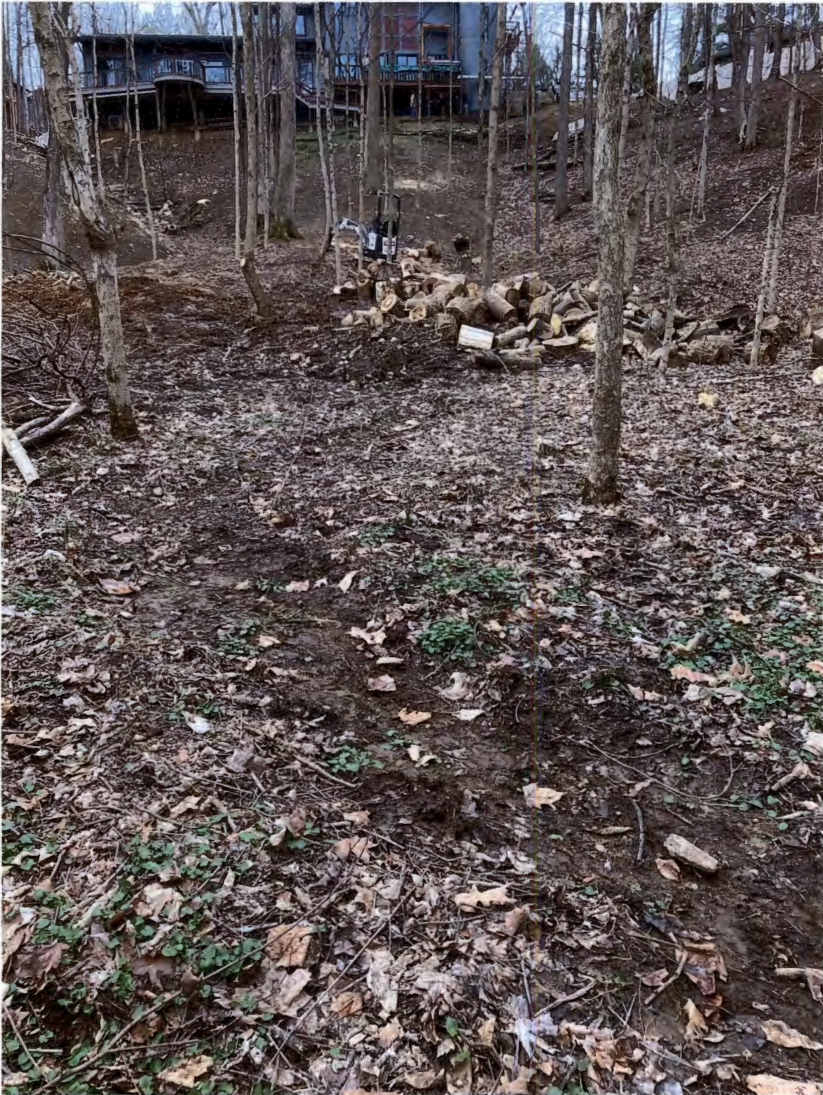
Photo 20: Sediment eroding off 2408 S Shadow Grove Ct from the disturbed land area downhill through to adjacent City-owned property and towards Jackson Creek 03/01/2024. Excavator still present on property.
