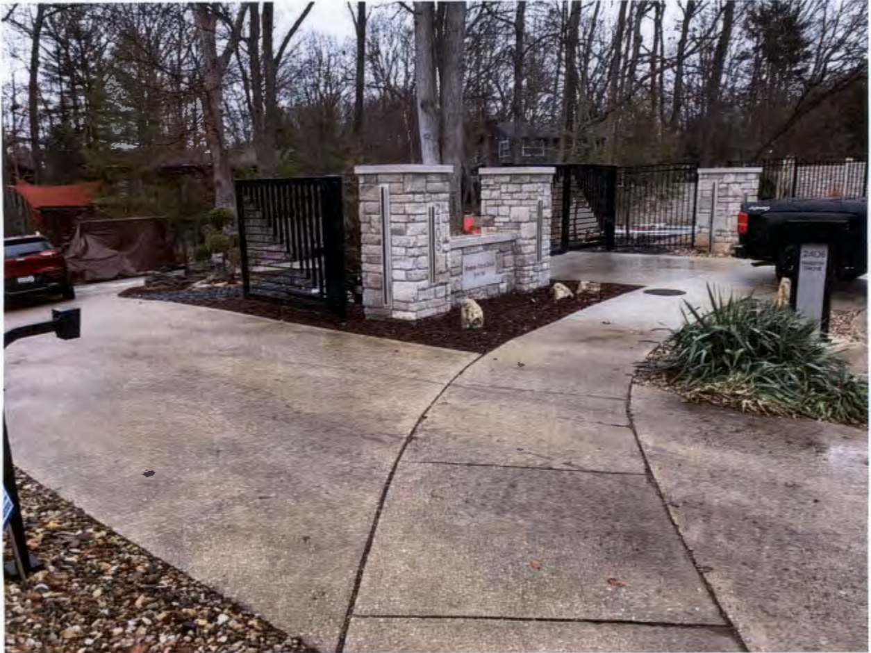
Photo 15: Multiple driveways in excess of the allowed number at 2408 S Shadow Grove Ct on 02/22/2024.
