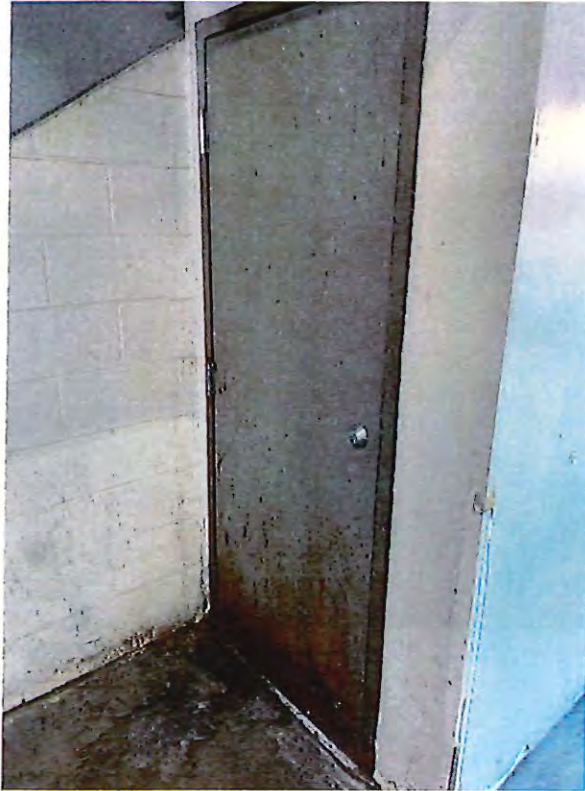
33 - door and frame corrosion.JPG
