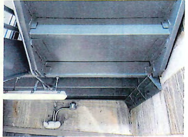
26 - east stair steel corrosion.JPG
