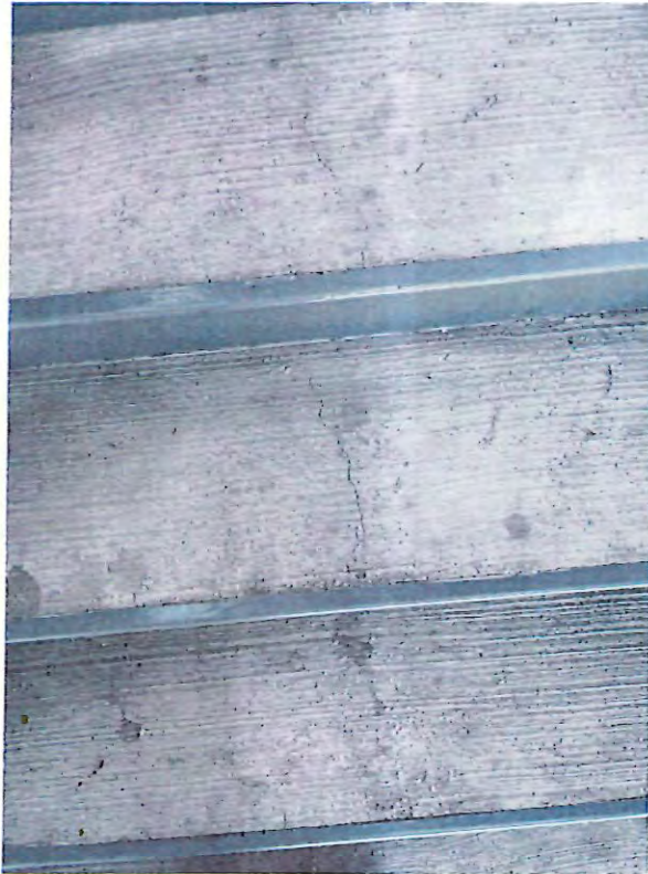
17 - crack in stair tread.JPG
