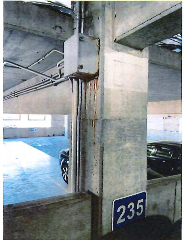
30 - corroded electrical box.JPG
