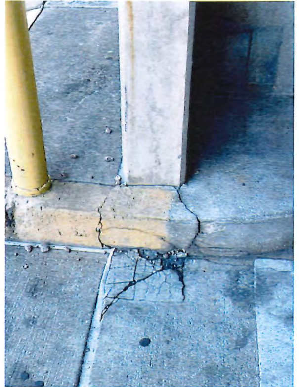
14 - spalled concrete curb.JPG
