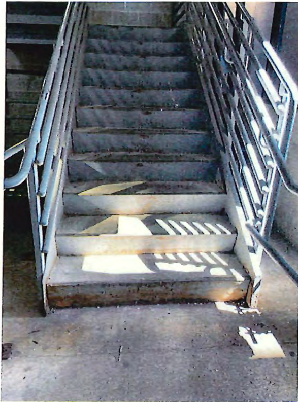
17 - stair steel corrosion.JPG
