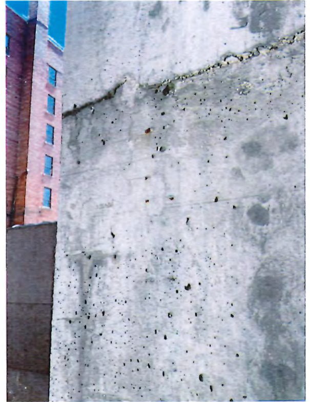
6 - column cracks with delamination.JPG
