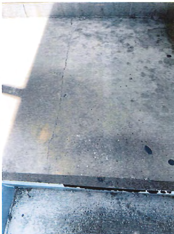
15 - crack in stair landing.JPG
