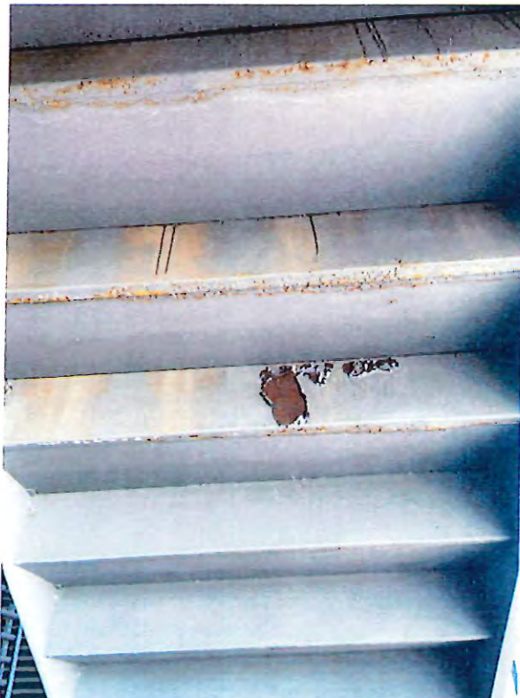
19 - stair steel corrosion.JPG
