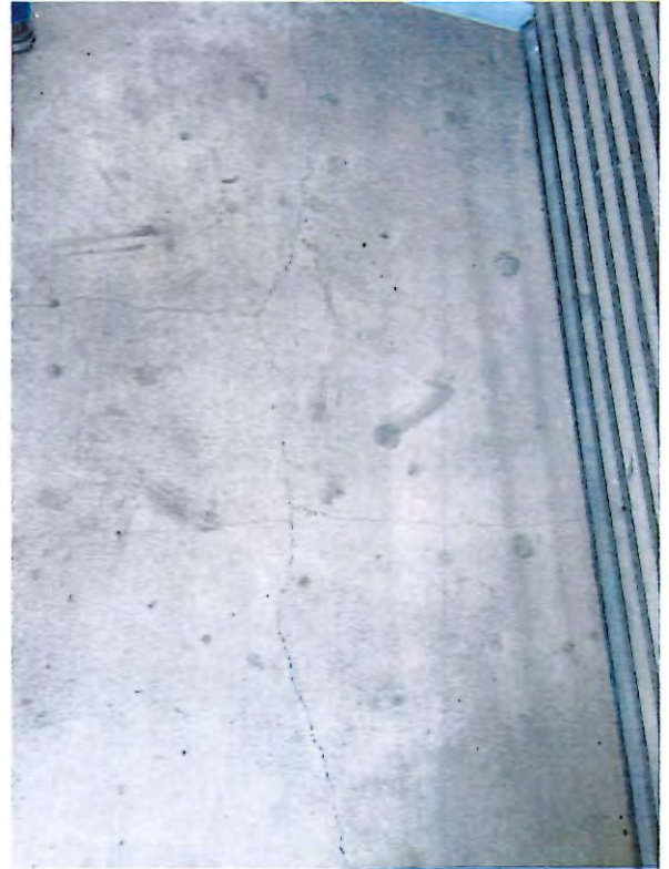
14 - crack in stair landing.JPG
