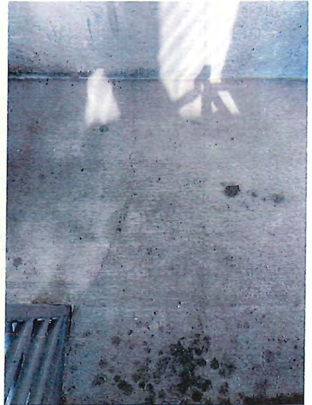
18 - crack in stair landing.JPG
