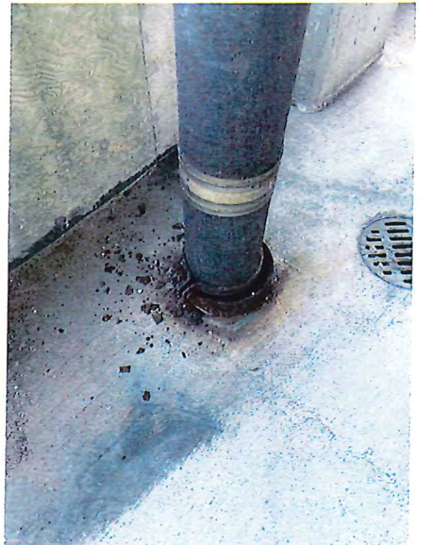
28 - corroded drain pipe sleeve.JPG
