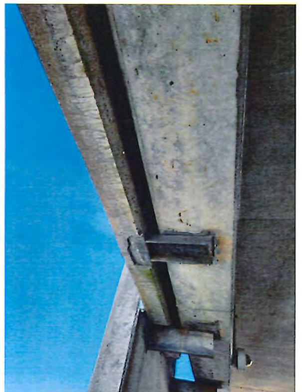
16 - spalled concrete at embed.JPG
