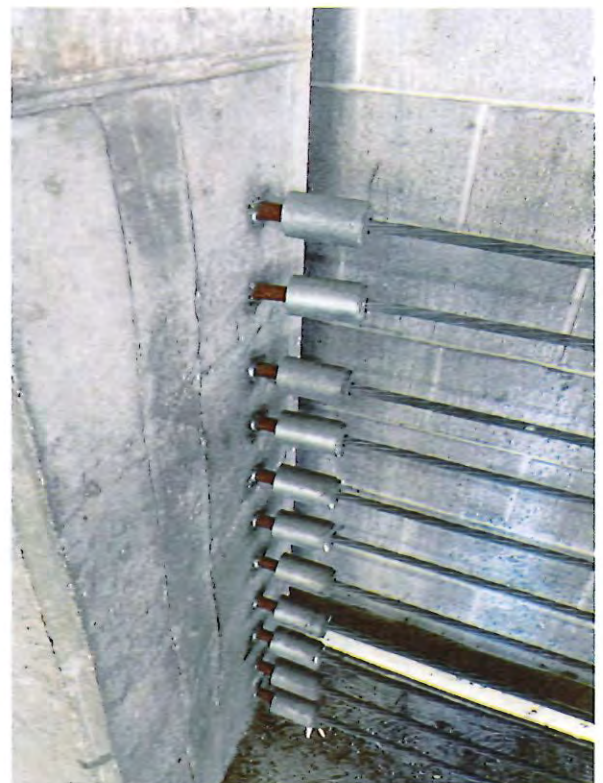
16 - corroded vehicular barrier cabling connection.JPG
