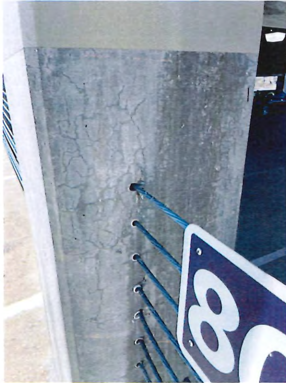
5 - column cracks with delamination.JPG
