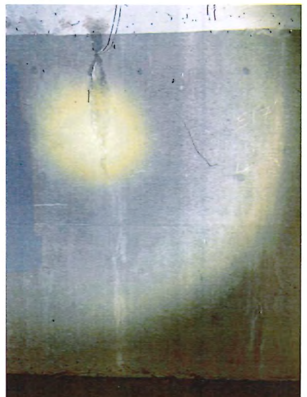
8 - basement level - wall crack.JPG
