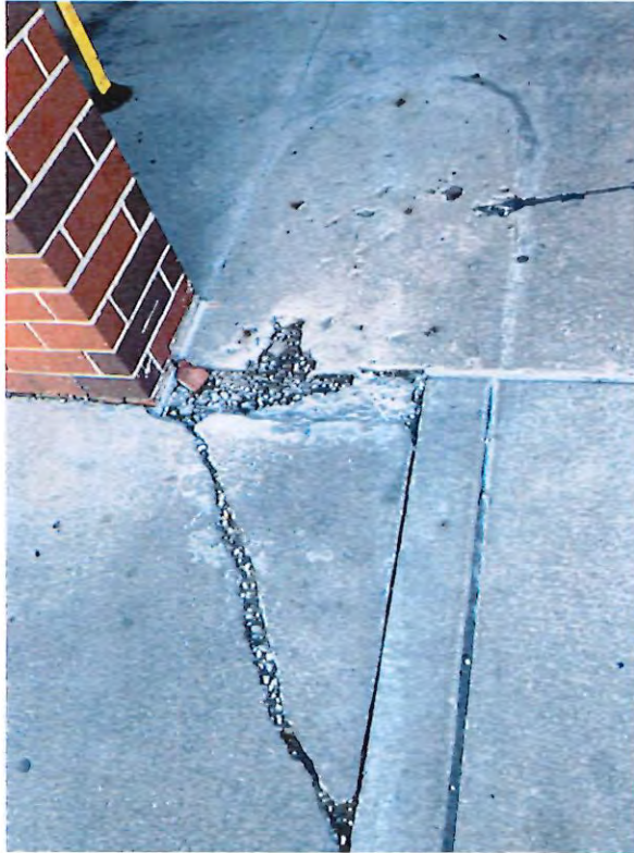
13 - SOG spalled concrete.JPG
