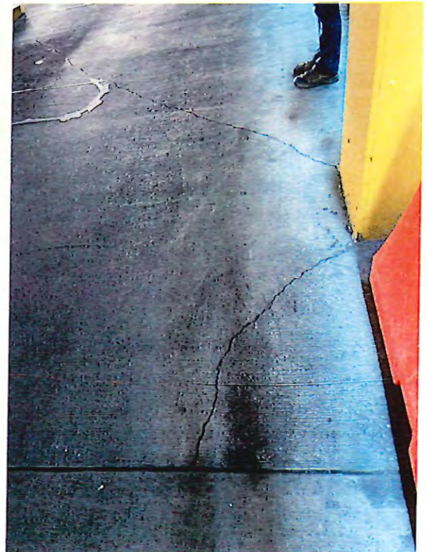
12 - SOG parking deck cracks.JPG
