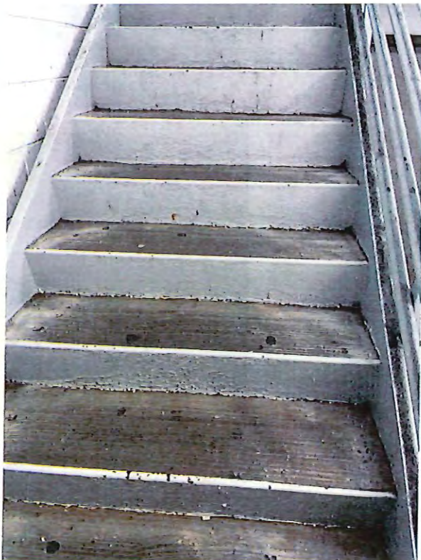
27 - west stair steel corrosion.JPG
