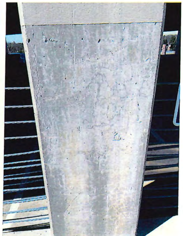
4 - column cracks with delamination.JPG
