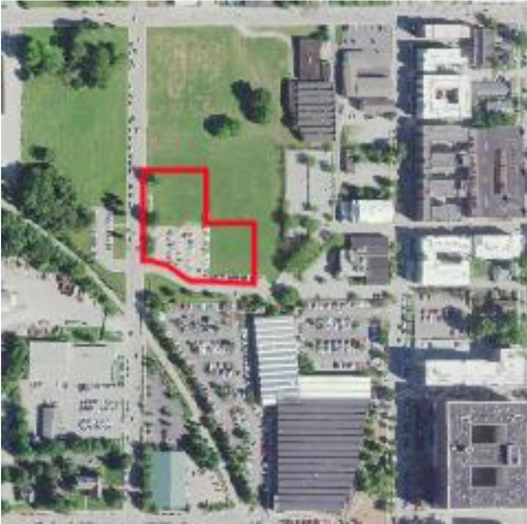
Trades District (2016): post-demolition of IU facilities
