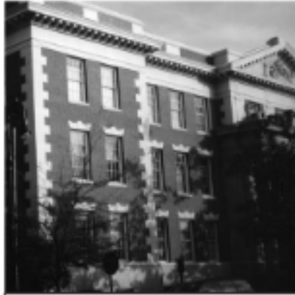
PHOTO: Ten years after being coated with ELASTOWALL 351 , limestone elements on this historic school retain a crisp, natural appearance.
