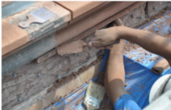
Custom SYSTEM 45 sandstone grade during trowel application at 21 Astor Place, NYC.
