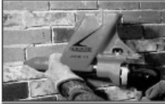
PHOTO: SPEC-JOINT 46 can be used in electric pointing guns without special admixtures or mix modification.
