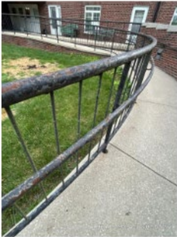
Handrails need repaired and repainted
