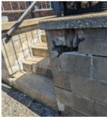
Failing Exterior Steps
