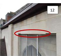
Stone lintel rotated downward over east side window near south end
