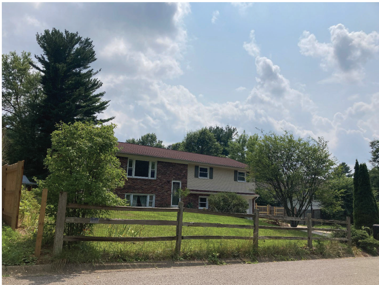
Photo 1: Fencing along the northern side of the property located in the public right-of-way and fencing along the eastern side of the property exceeding the allowed height at 4216 E Penn Ct on 07/25/2024.
