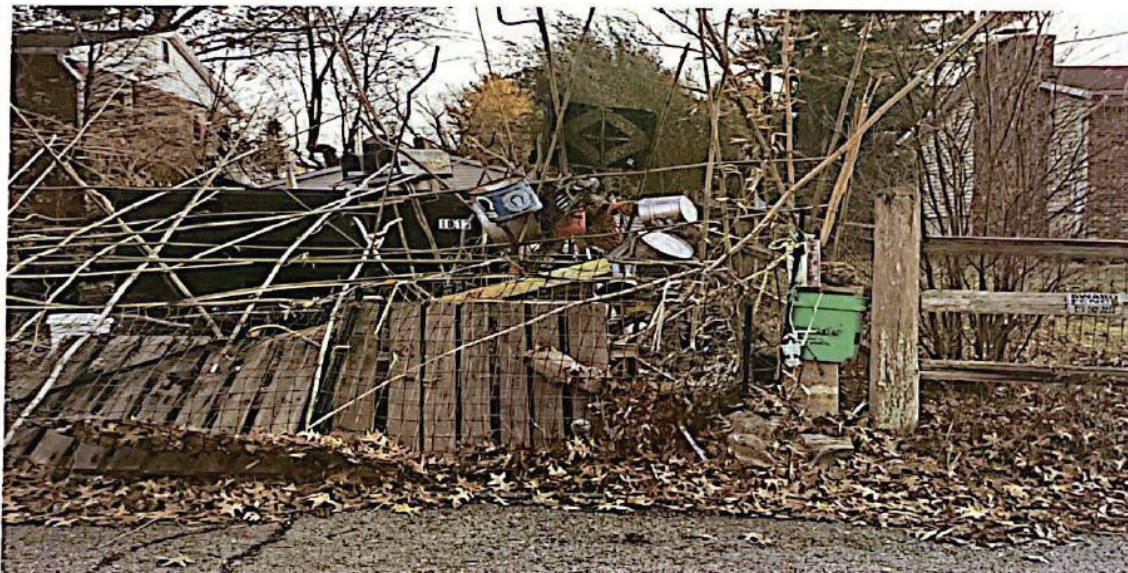
Previous fence structure (right) which deteriorated over time due to the property owner adjacent to 4216 East Penn Court placing heavy objects leaning on the fence (left)
