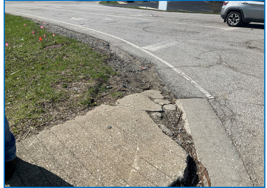
Photo 6 – View of deteriorated concrete curb at the southeast quadrant of the SR 45 and Liberty Drive/South Hickory Leaf Drive intersection (04/01/2025).
