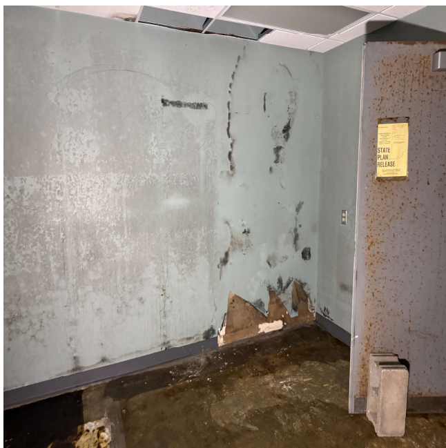
Photo 3: Biological growth behind vinyl cove base traveling up wall - August 2025
