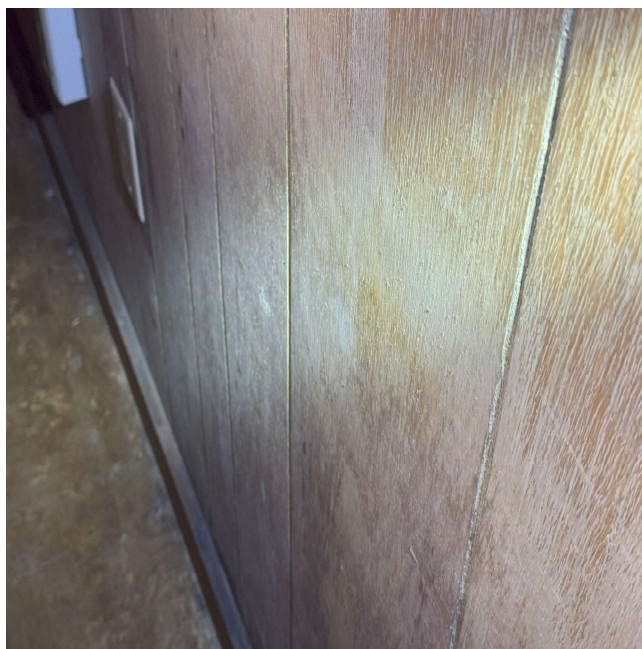
Photo 4: Biological growth on wood paneling on first floor
