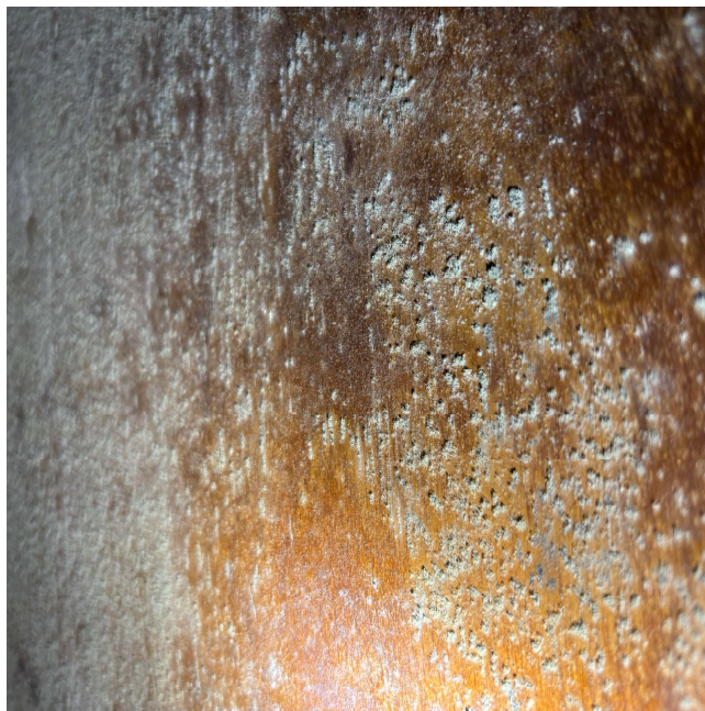
Photo 2: Biological growth with fruiting structures on wooden door on first floor - August 2025
