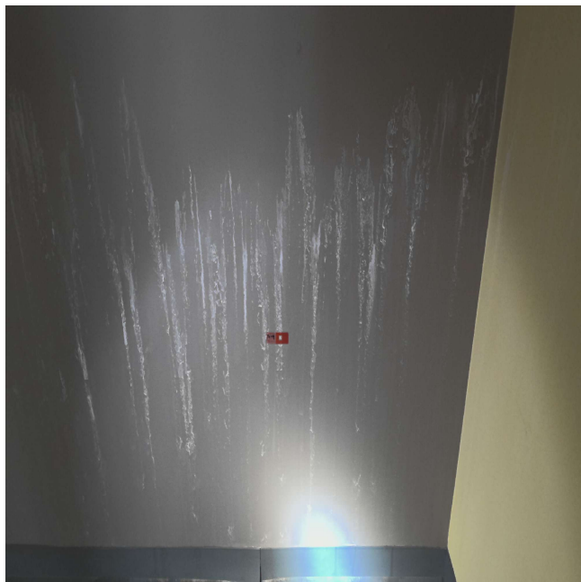
Photo 1: Water damage behind vinyl cove base on fourth floor - August 2025
