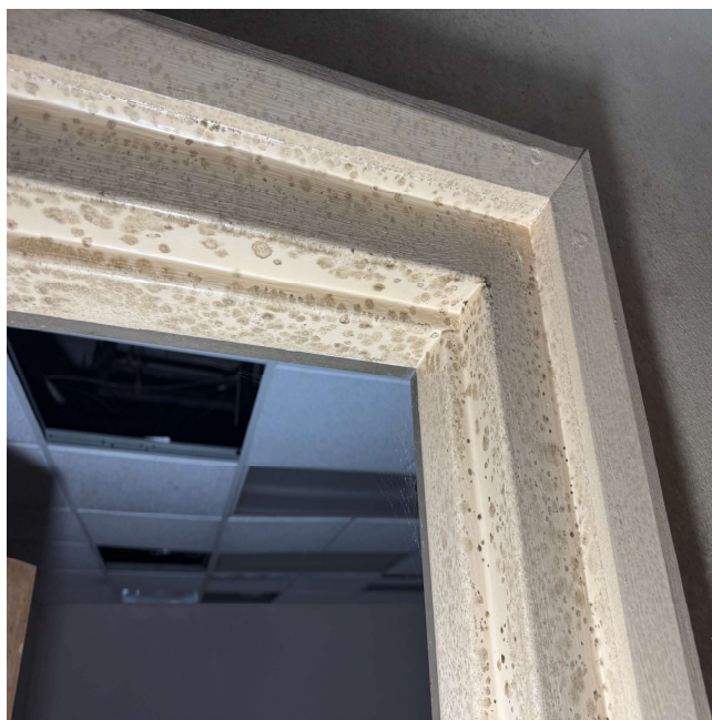
Photo 4: Biological growth on painted metal on first floor - August 2025
