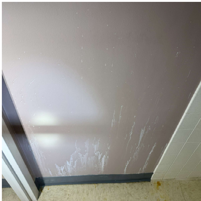
Photo 1: Water damage behind vinyl cove base on fourth floor
