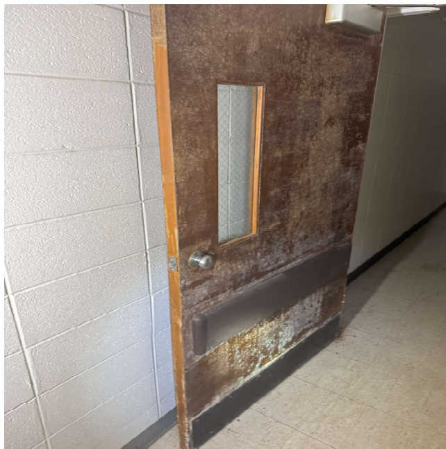
Photo 2: Biological growth on wooden door on first floor
