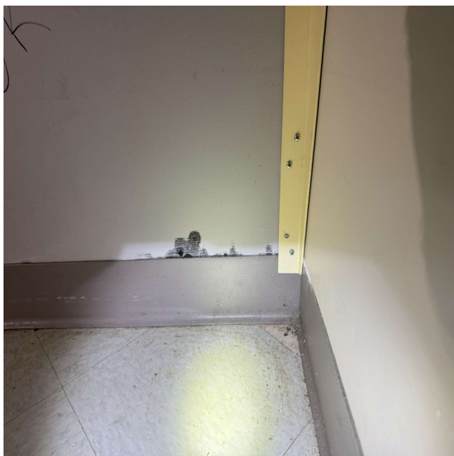
Photo 3: Biological growth behind vinyl cove base on fourth floor
