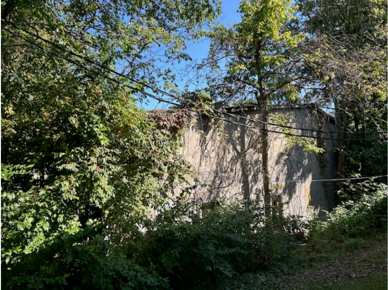
Shed as seen from N Fairview St
