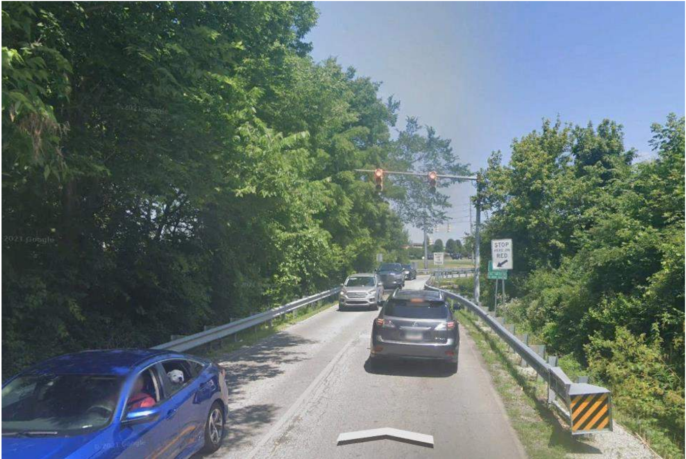
Figure 2 Example of Signal Controlled Single Lane Bridge
