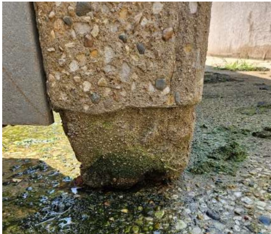
Figure 6 Concrete spall/wear at base of north end of interior wall
