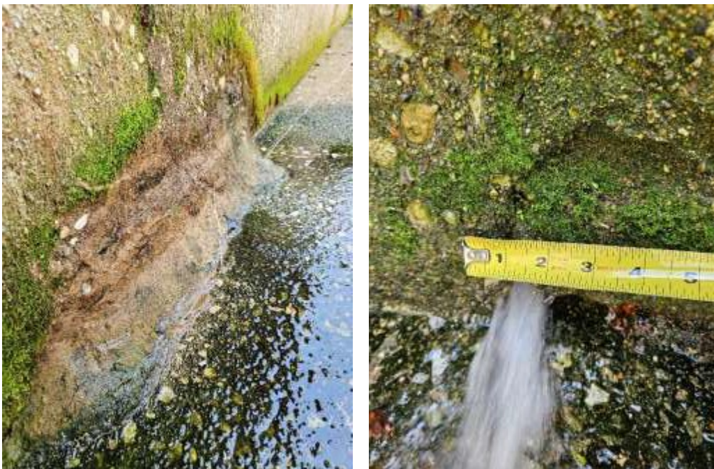
Figure 3 Holes spraying water in contact basin no. 1 (left: pinholes; right: large hole)
