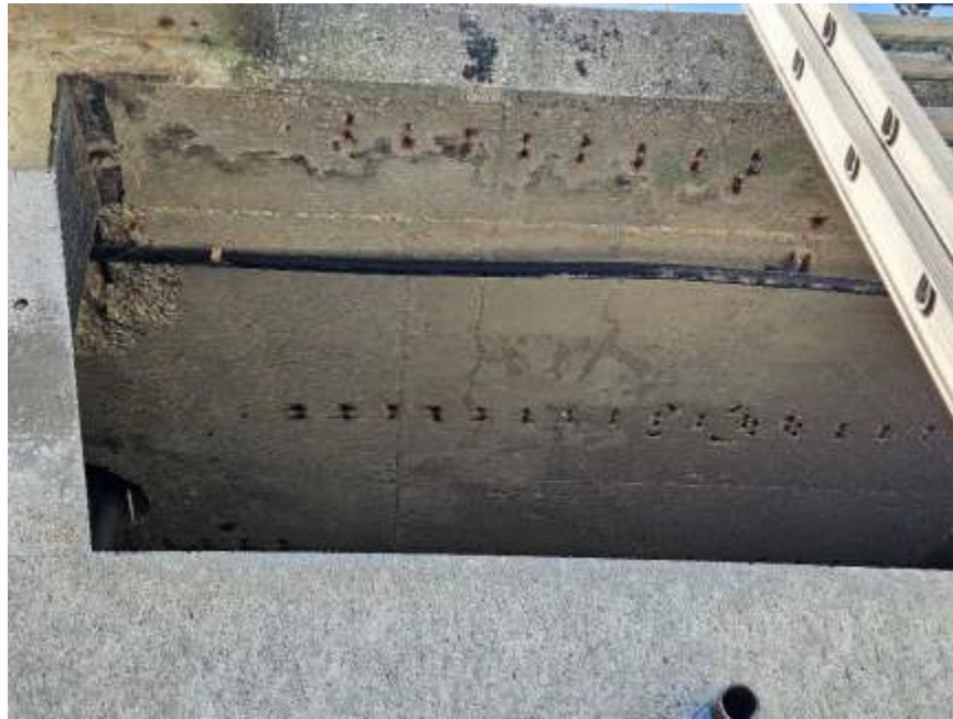
Figure 5 Concrete spall and exposed reinforcing steel on underside of deck over effluent outfall
