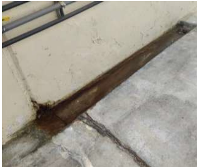
Figure 9 Active Leak Through an Expansion Joint in the Basin Complex
