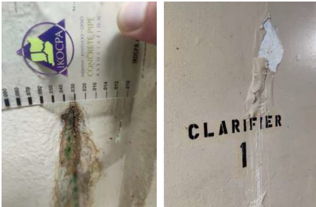
Figure 4 Examples of cracks in basin complex (left: wide crack; right: representative crack)
