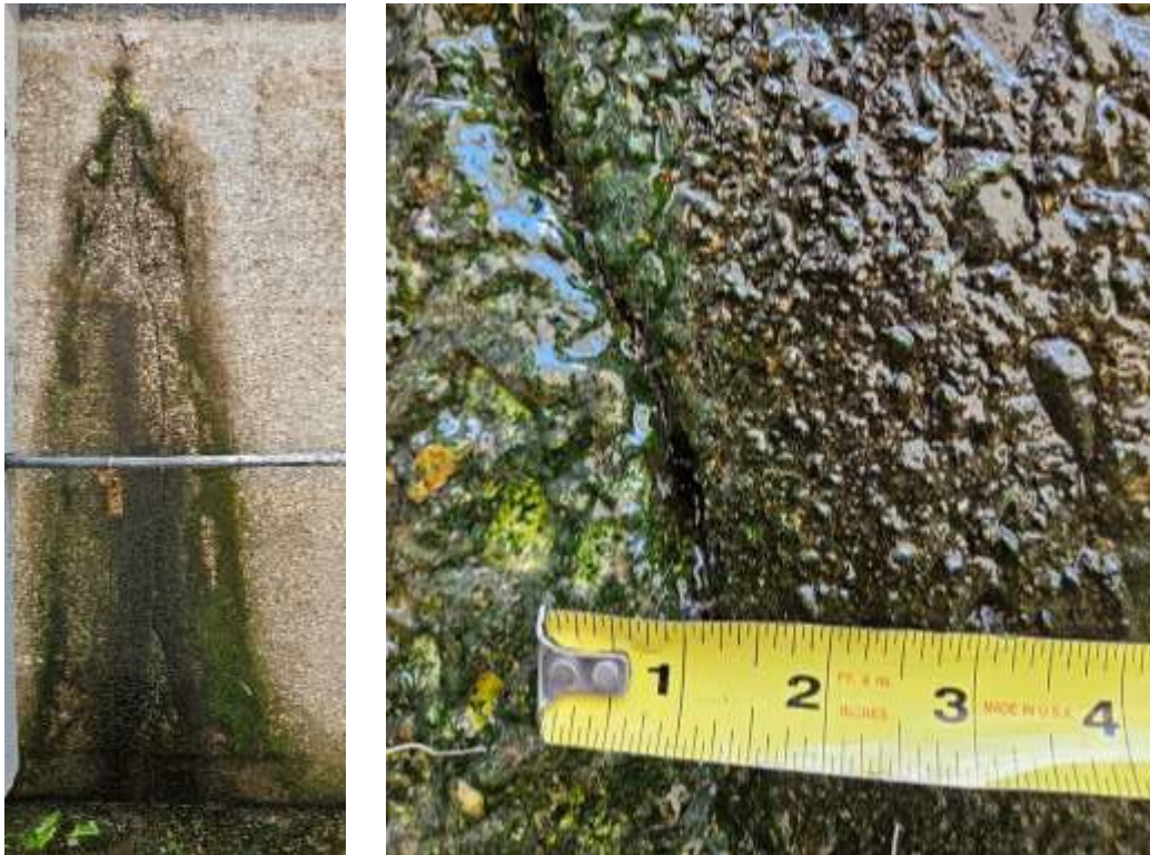
Figure 2 Examples of cracks in contact basin no. 1 (left: full length of crack; right: close-up)
