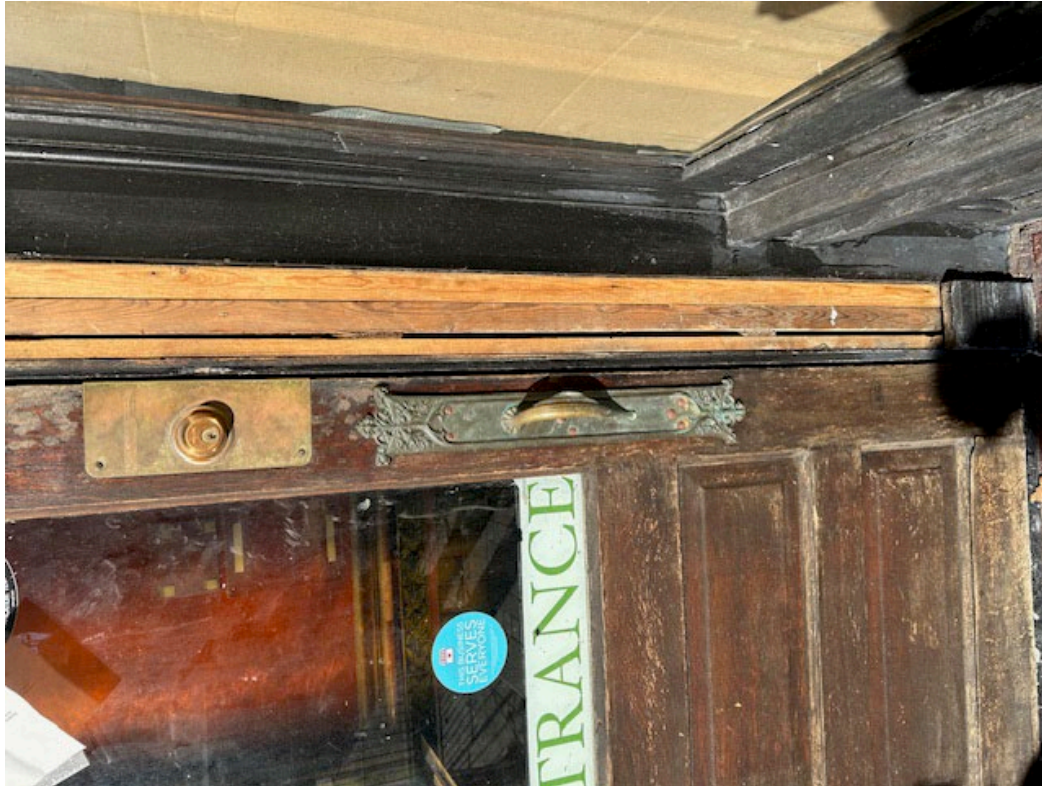
2x4s installed for vestibule
