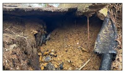
Figure 5: Seepage Under Spillway Chute
