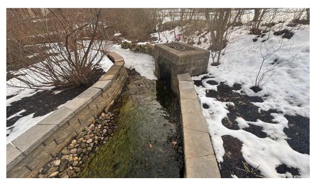
Figure B25: Entrance to culvert under E. St. Remy Dr. that conveys main tributary to reservoir
