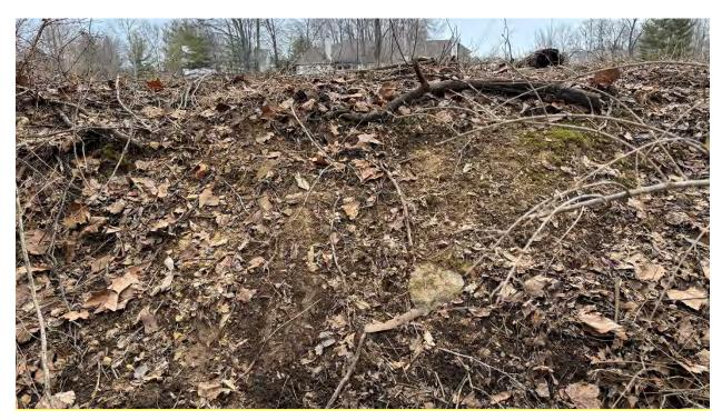
Figure B11: Downstream slope of embankment (Note: exposed coarse soils and rock)
