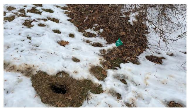
Figure B4: Rodent activity and/or sinkhole on upstream slope near sanitary sewer
