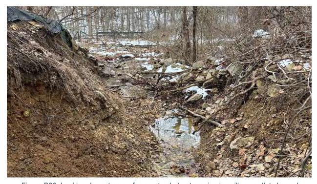
Figure B20: Looking downstream of concrete chute at erosion in spillway outlet channel
