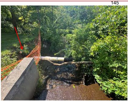
Photopoint 15 – Looking east along UNT2 to Jackson Creek from the spillway. Note the extreme erosion (red arrow).
