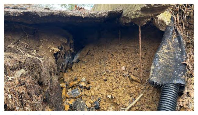
Figure B18: End of concrete chute for spillway looking upstream at undermined portion
