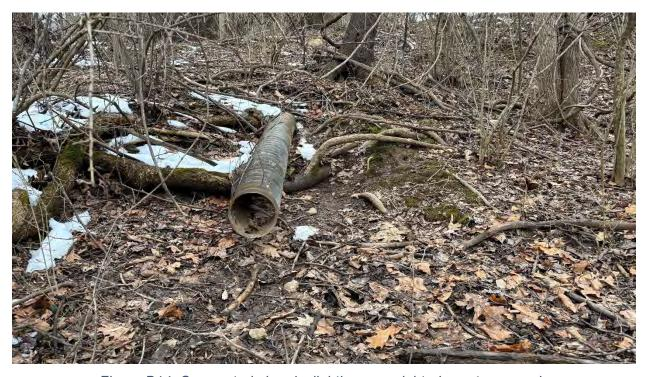
Figure B14: Corrugated pipe daylighting near right, downstream groin
