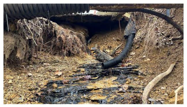
Figure B19: Undermining of concrete chute for spillway (Note: exposed drainage pipe)
