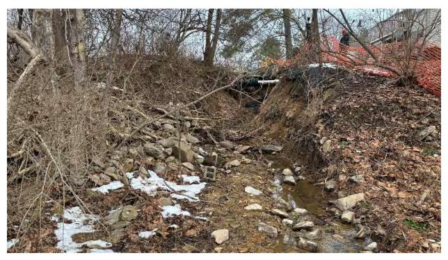
Figure B21: Looking upstream at eroded outlet channel with concrete chute in background
