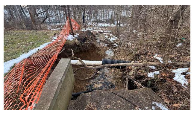
Figure B17: End of concrete chute for spillway (Note: erosion and exposed sanitary sewer)
