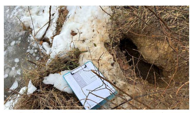
Figure B3: Rodent activity and/or sinkhole on upstream slope near edge of water
