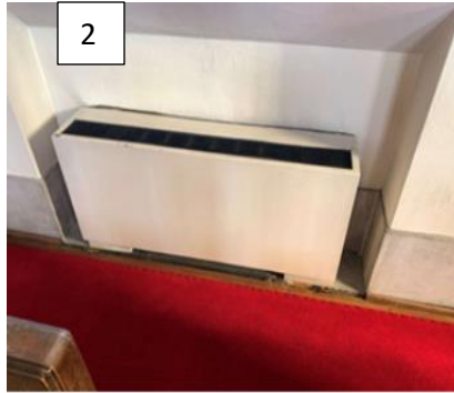
Figure 20: Sanctuary Fan Coil Unit (Exposed)
