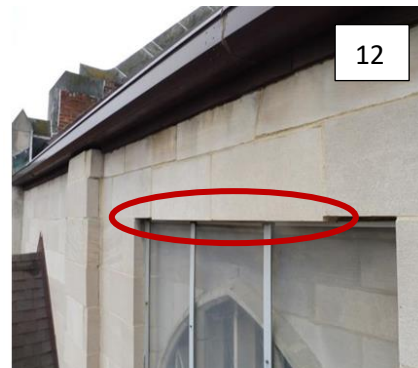
Stone lintel rotated downward over east side window near south end.
