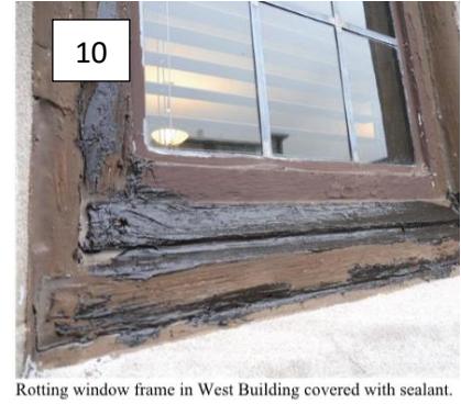
Rotting window frame in West Building covered with sealant.
