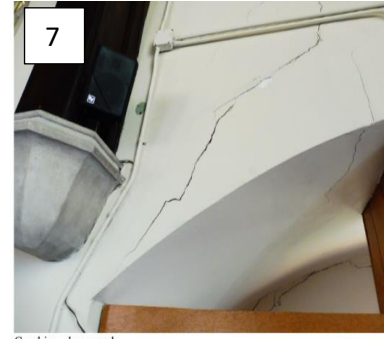
Cracking above arch.
