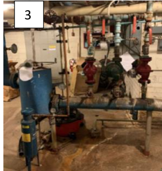
Figure 8: Heating Water System Pumps
