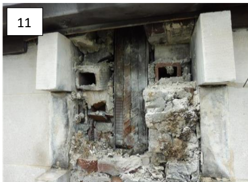
Outer portion of rubble infill removed to expose unprotected wood end of roof!
