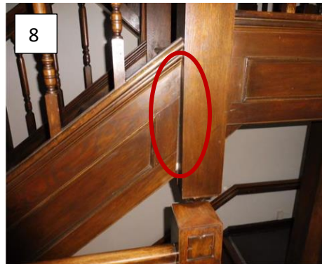
Failed mortise and tenon joint of stair stringer.
