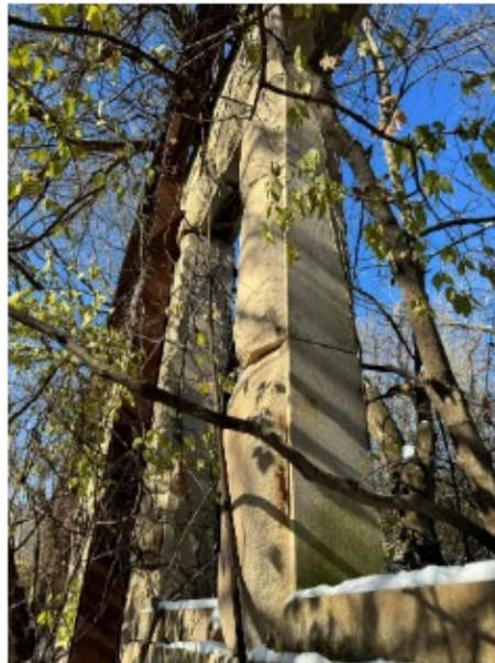
Photo 8: Limestone Column Blocks
