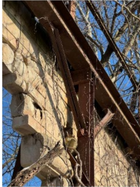
Photo 9: Steel Frame Details
