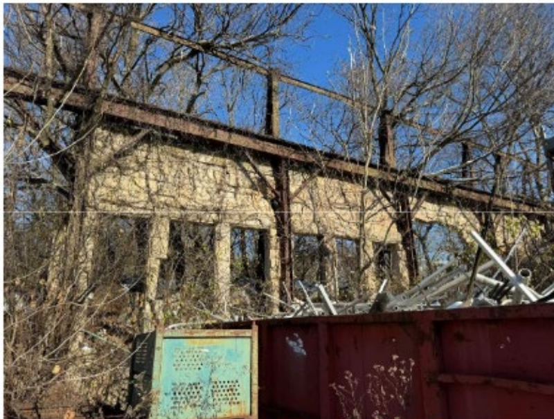
Photo 2: South Face of Wall, West End (Looking North)
