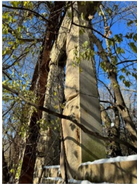
Photo 8: Limestone Column Blocks
