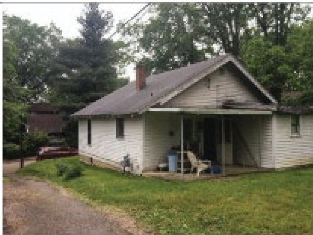
South Elevation, looking west along alley
