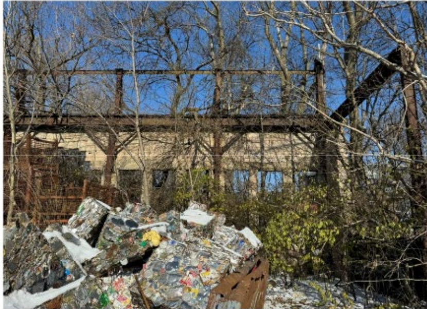
Photo 3: South Face of Wall, East End (Looking South)
