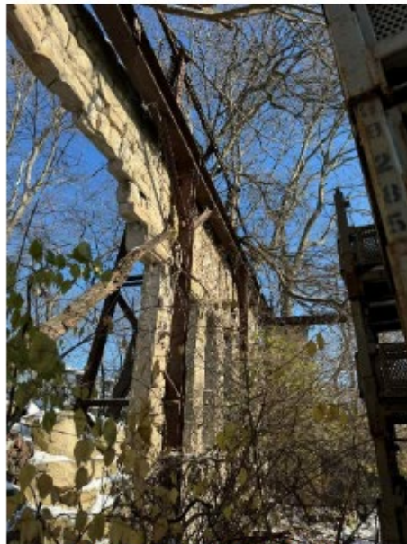
Photo 10: Steel Frame Support Details
