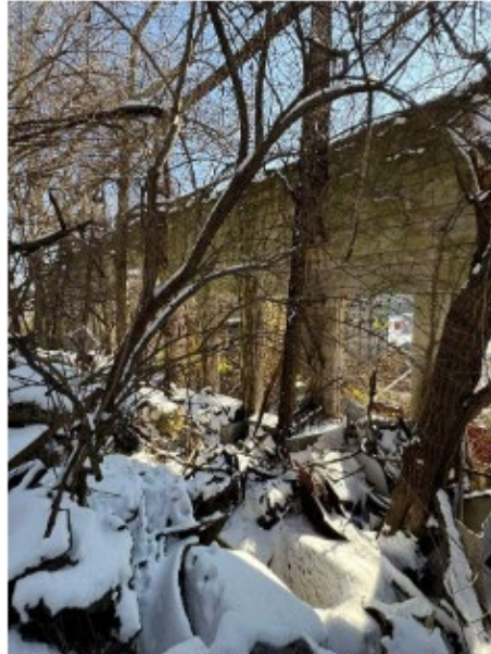
Photo 5: North Face of Wall, West End (Looking Southeast)
