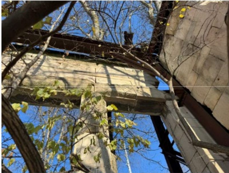
Photo 7: Limestone Wall with Limited Connection to Steel Frame
