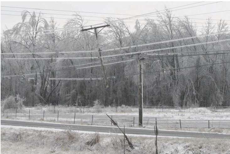
Figure 47 Ice Covered Power Lines
