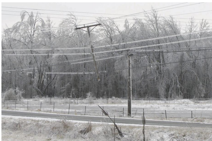
Figure 47 Ice Covered Power Lines
