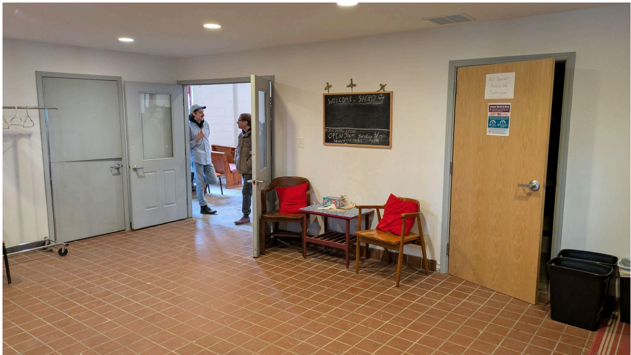
Lobby - West Wall
