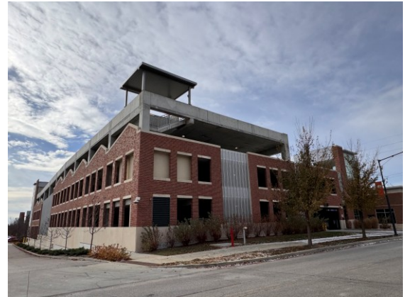
Trades District garage at W. 10 th Street
