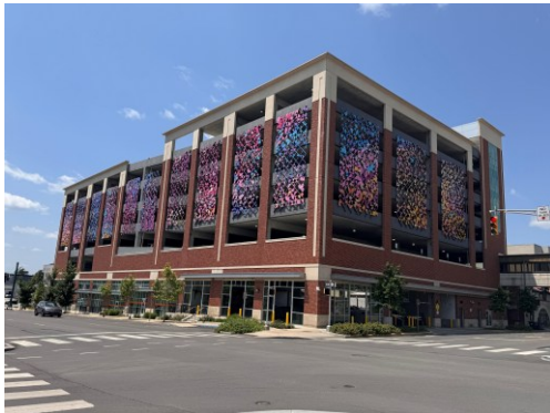
Art installation on façade of 4 th Street garage, but no clear signage indicating public parking from College Ave.
