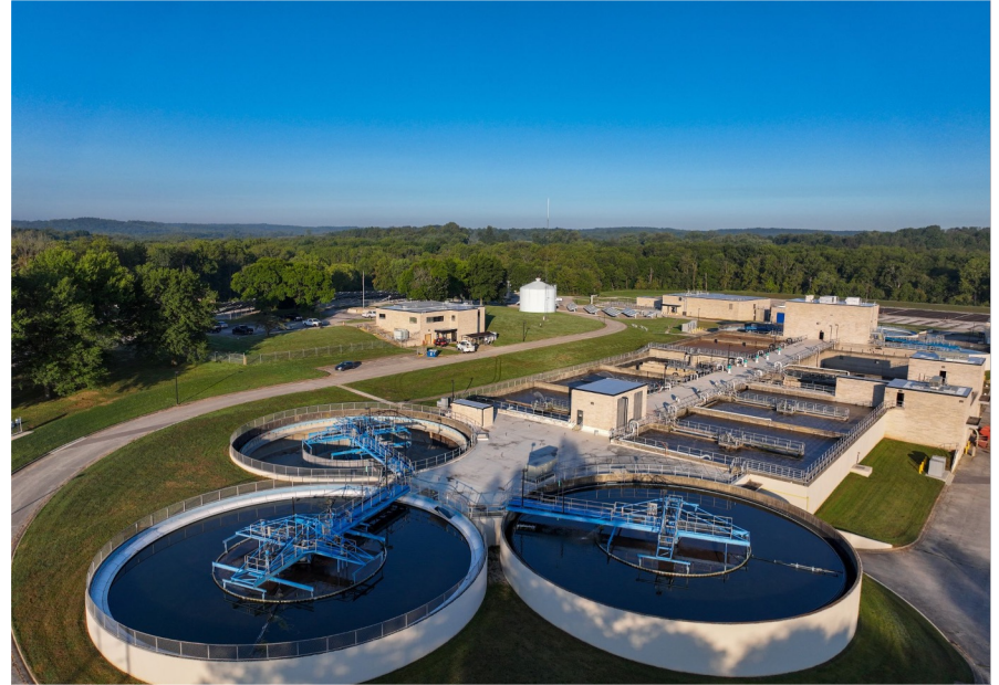
Dillman Wastewater Treatment Plant
