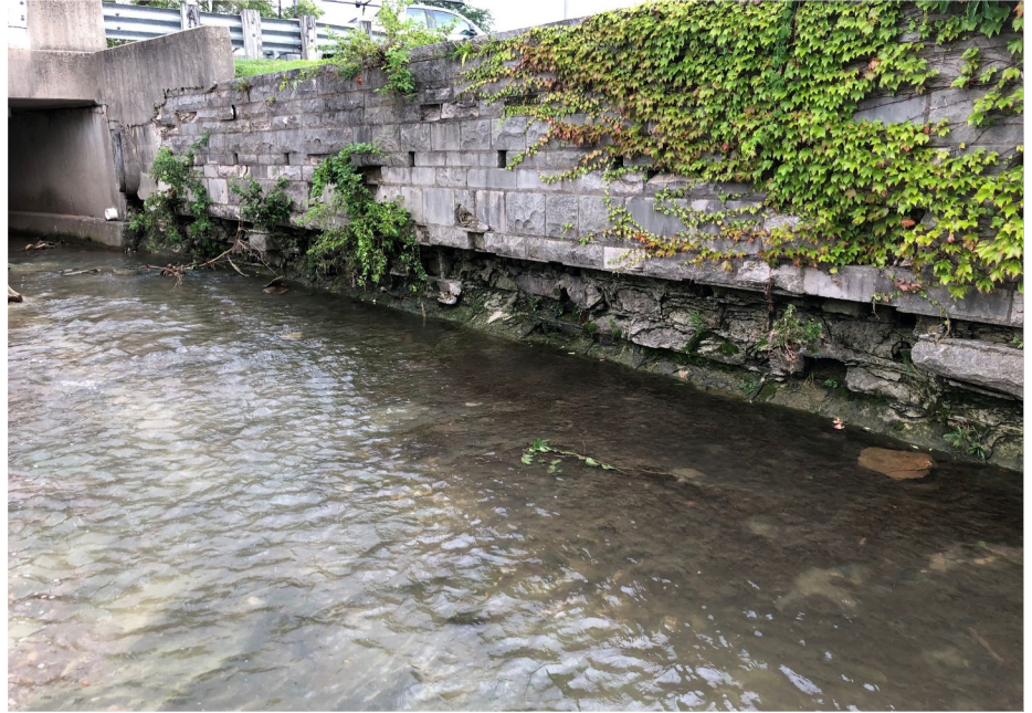
Clear Creek Stormwater Channel
