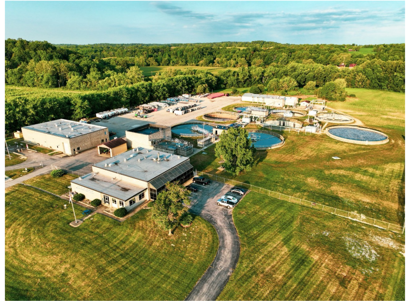
Blucher Poole Wastewater Treatment Plant
