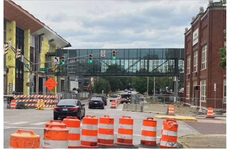
S College Avenue Temporary Closures
