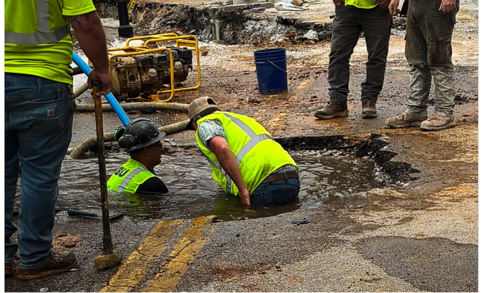
T&D Crew working on West 2nd Street Modernization project.
