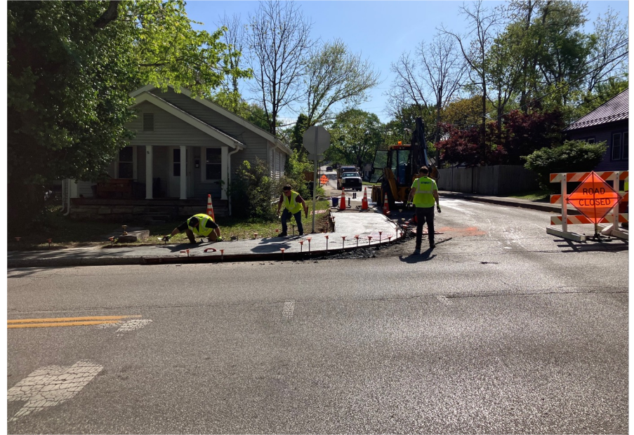
ADA-compliant curb ramp installed
