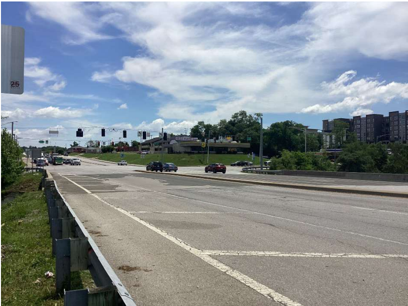
3: Looking southeast along the westbound lane of SR 45, in the middle of the project area.
