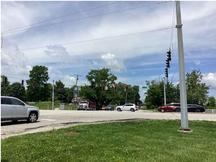
10: Looking northwest across the intersection of N. Kinser Pike and SR 45, southwest quadrant.
