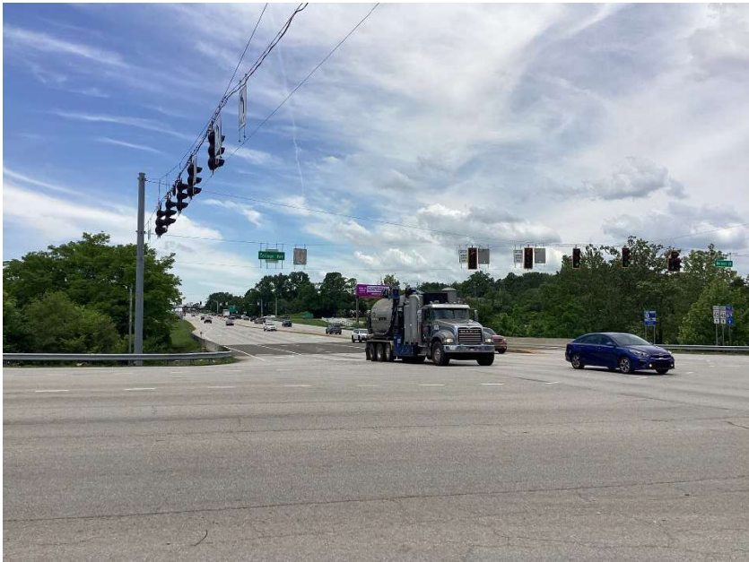
8: Looking west across the intersection of N. Walnut Street and SR 45, southeast quadrant.
