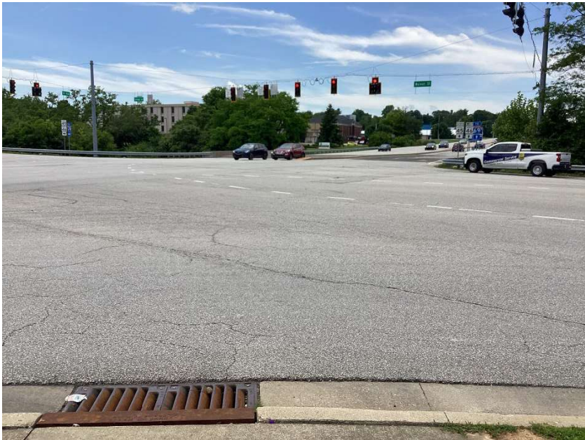
6: Looking southwest across the intersection of N. Walnut Street and SR 45 nearing the end of the project area, northeast quadrant.
