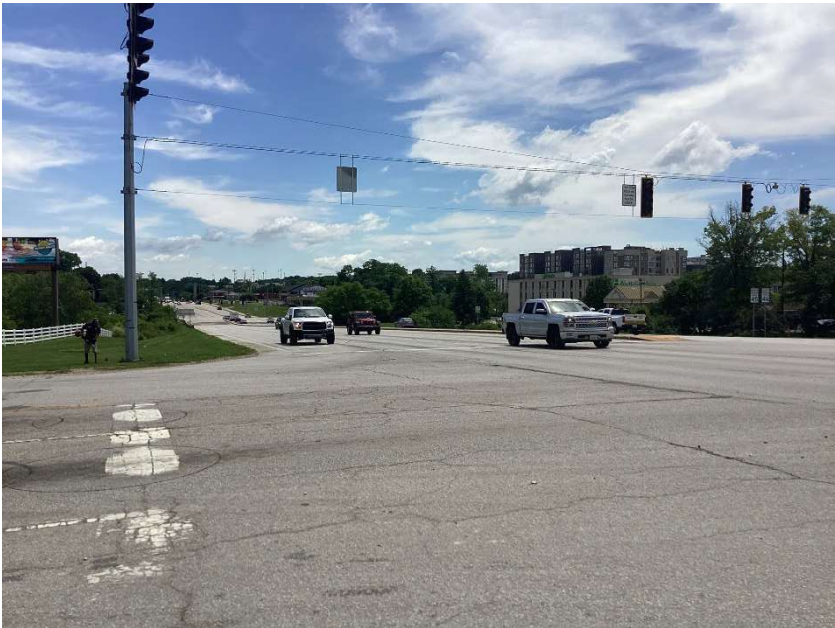
1: Looking southeast along the eastbound lane of SR 45, at the start of the project area, in the northeast quadrant.
