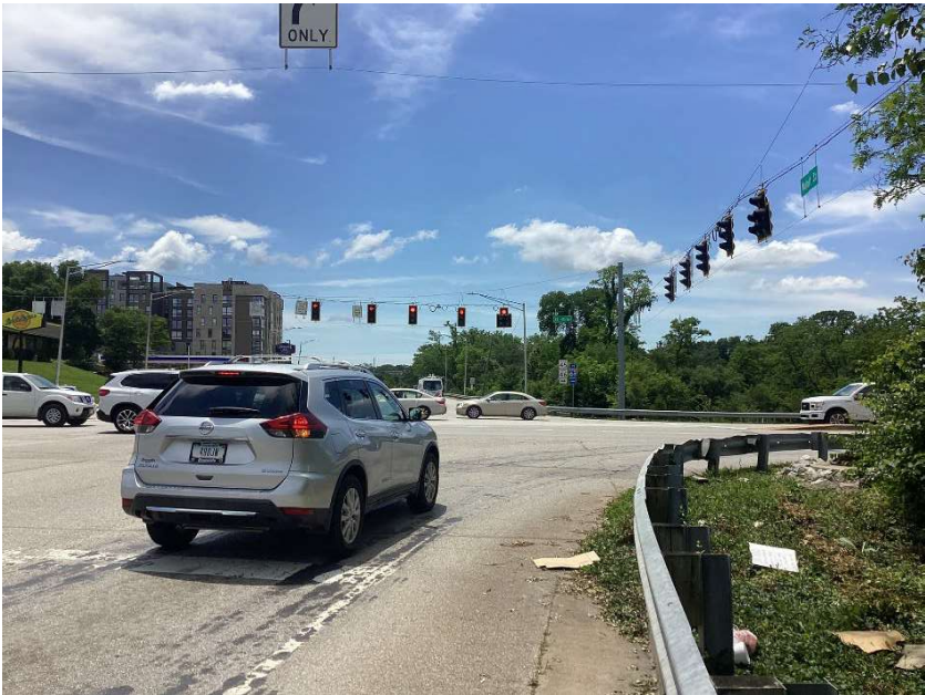
5: Looking south at the intersection of N. Walnut Street and SR 45 nearing the end of the project area, northeast quadrant.
