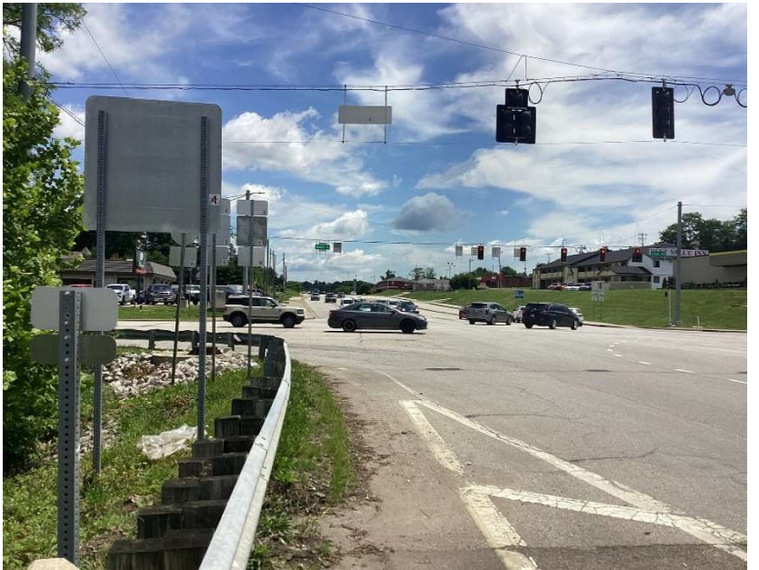
4: Looking east along the westbound lane of SR 45 nearing the end of the project area.
