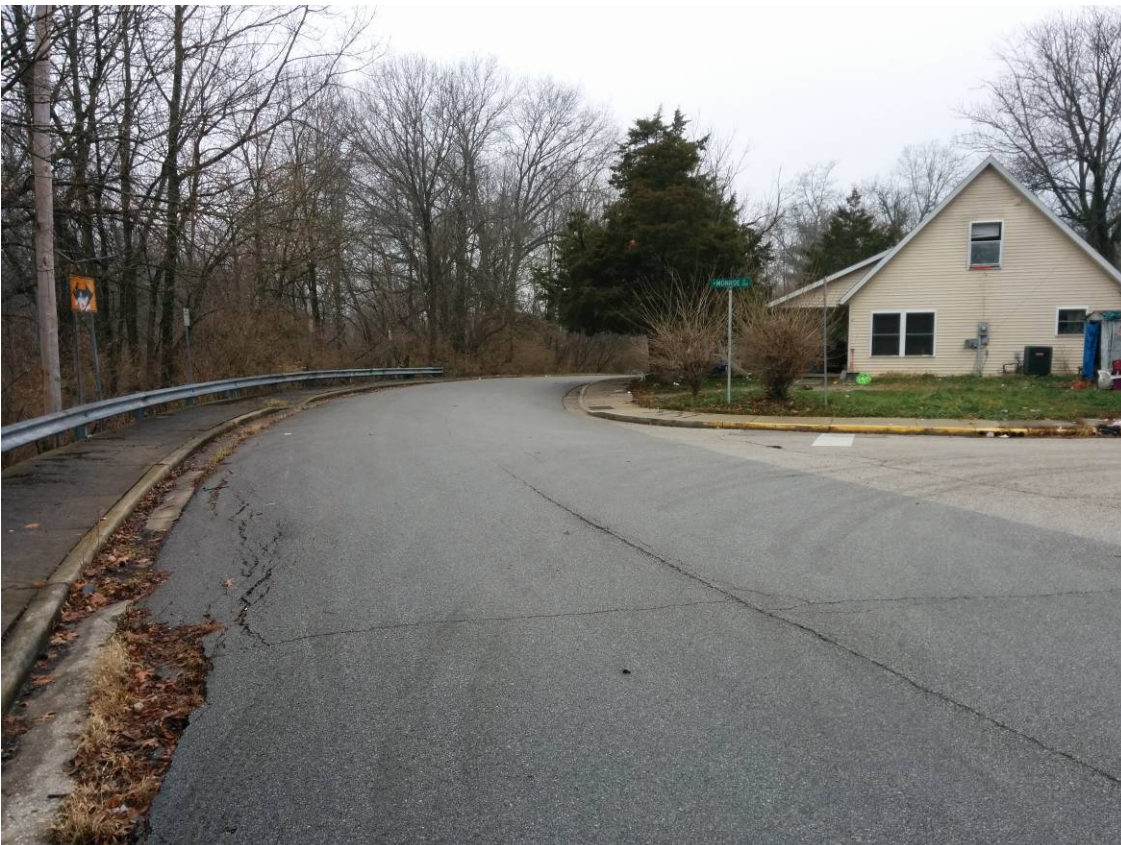
10 th Street looking west towards Monroe Street (~25 feet wide)
