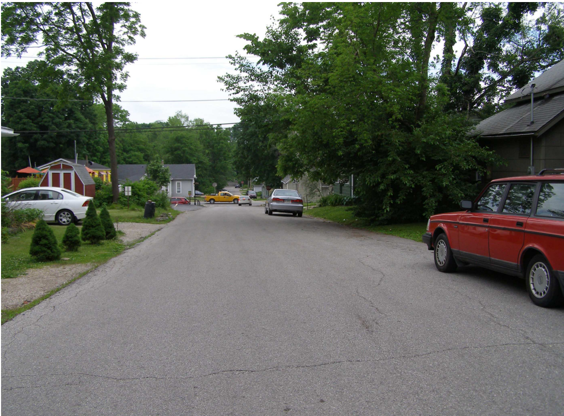
N. Fairview Street (~22') looking southbound towards the alley and W. Kirkwood Avenue.
