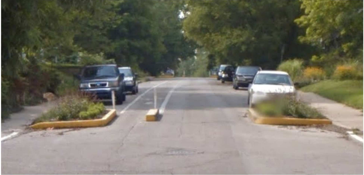
(Washington Street traffic bump-outs – photo provided by Mr. Brosner)
