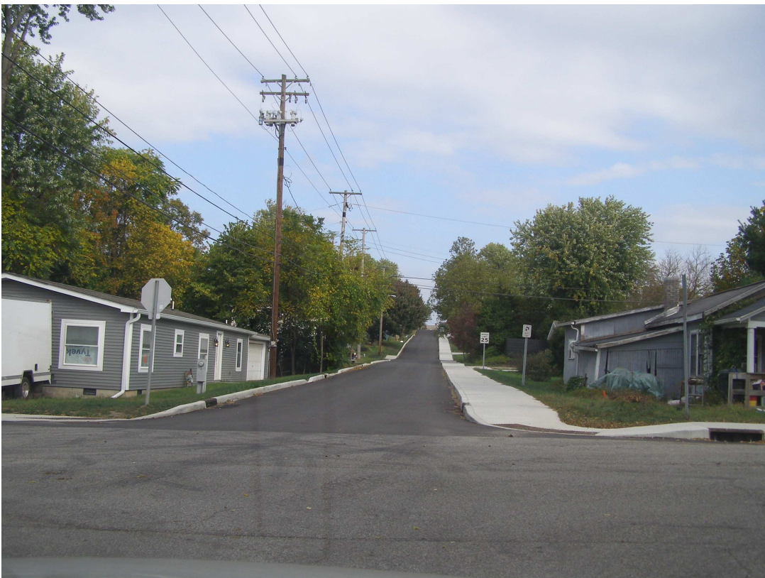
Looking north along S. Fairview Street from Allen Street (~24); new curbs on both sides of street, plus new sidewalk.
