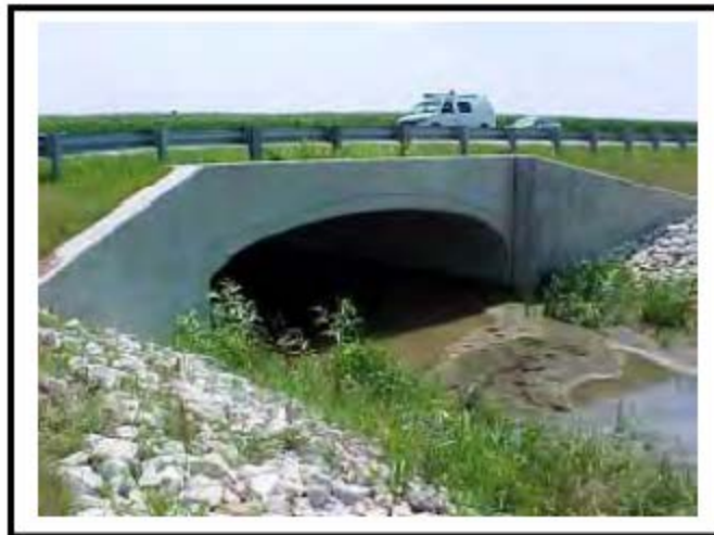
Figure 1:6-5: Precast Concrete Underfill Bridge
