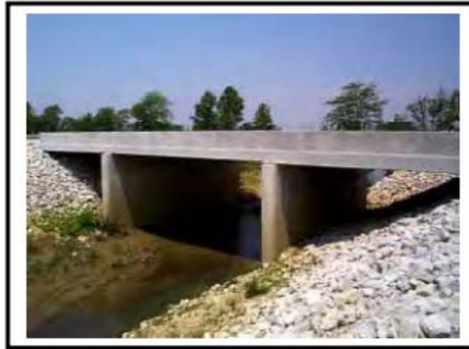
Figure 1:6-4: Continuous Reinforced Concrete Slab Bridge
