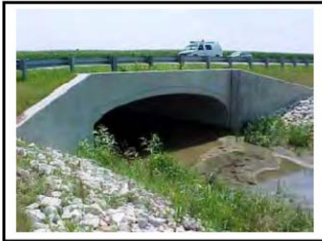
Figure 1:6-5: Precast Concrete Underfill Bridge
