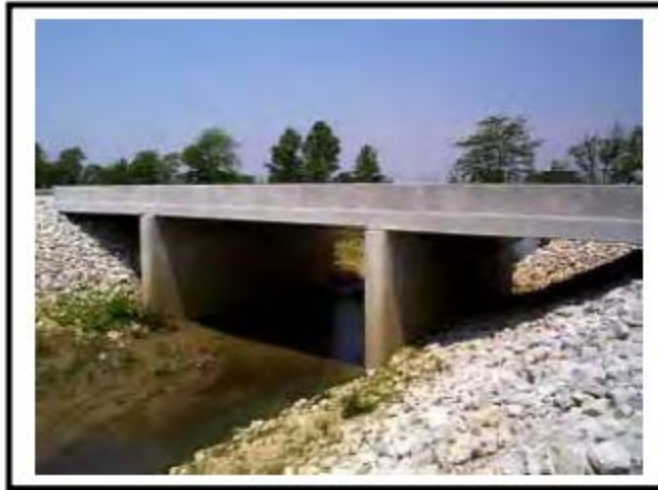
Figure 1:6-4: Continuous Reinforced Concrete Slab Bridge
