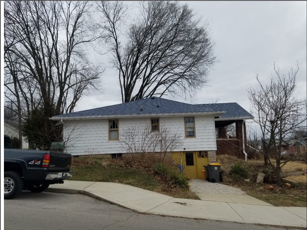
West side of house showing west facing planes of the roof that will have solar panels. View from Fairview Street lookin east.
