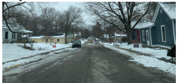
The above photo shows 6th St. between 1st alley east of Oak St. and Oak St. from west to east
