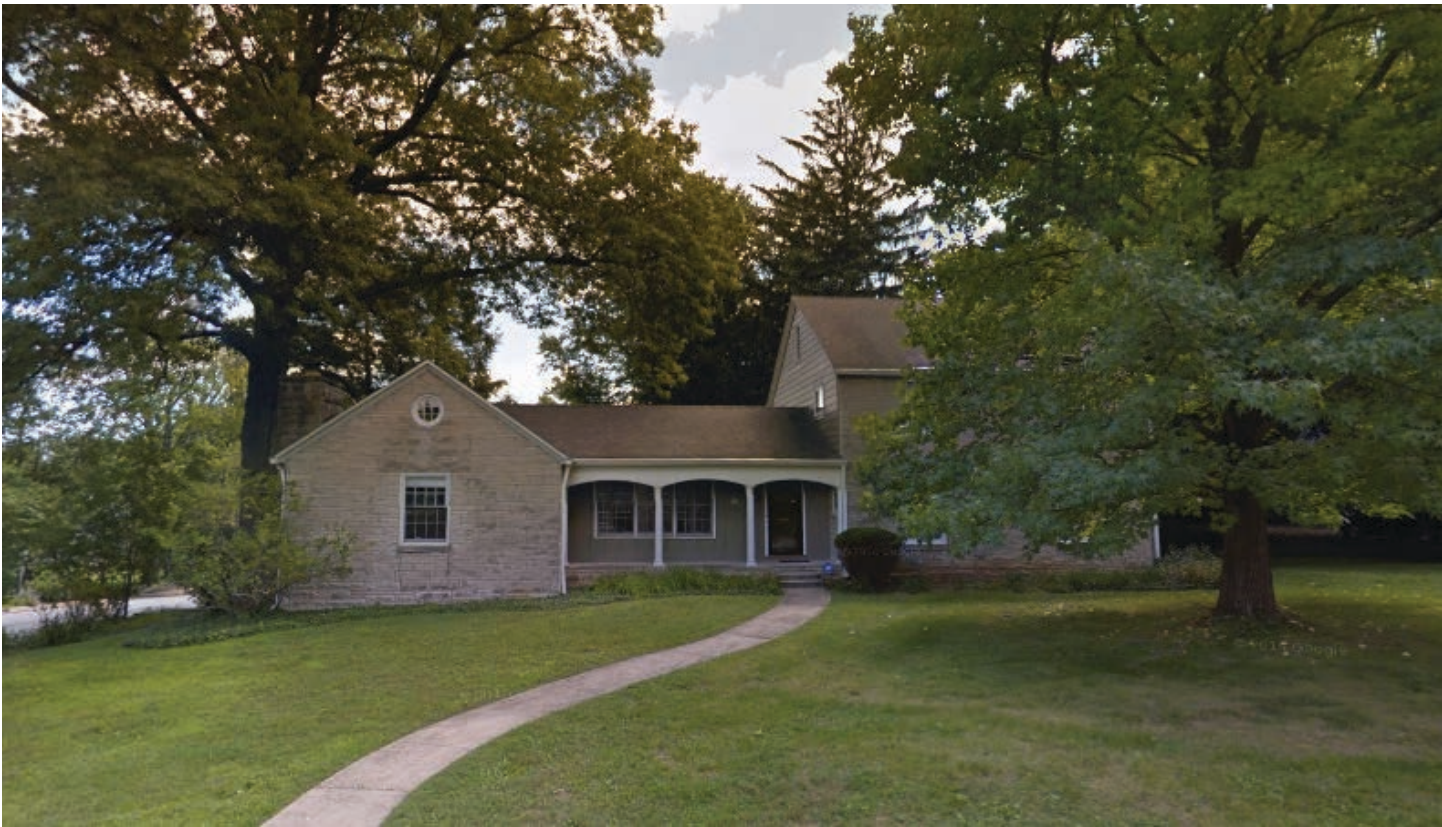
Front of Building towards Ballantine Rd
