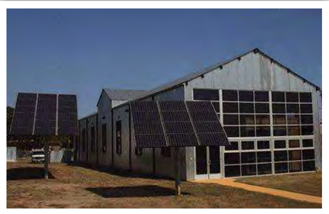
Recommended Free-standing solar panels have been installed here that are visible but appropriately located at the rear of the property and compatible with the character of this industrial site.
