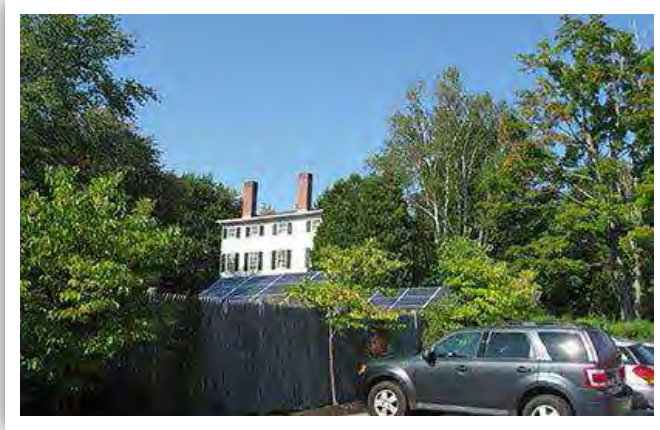
Not Recommended Although installing solar panels behind a rear parking lot might be a suitable location in many cases, here the panels negatively impact the historic property on which they are located.
