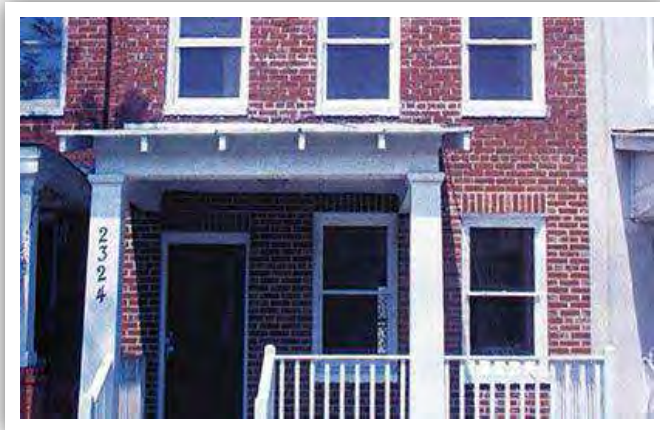
Recommended Solar panels were installed appropriately on the rear portion of the roof on this historic row house that are not visible from the primary elevation.
