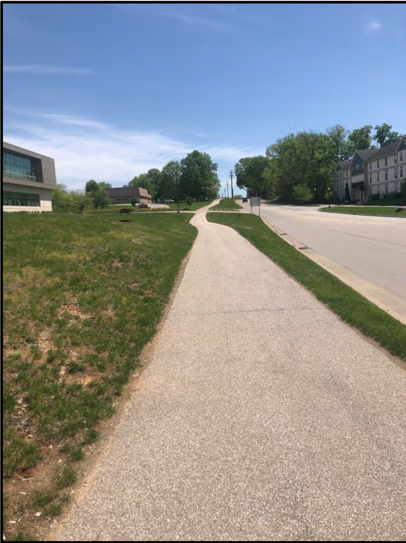
5. View east along SR 45. 5/4/2020
