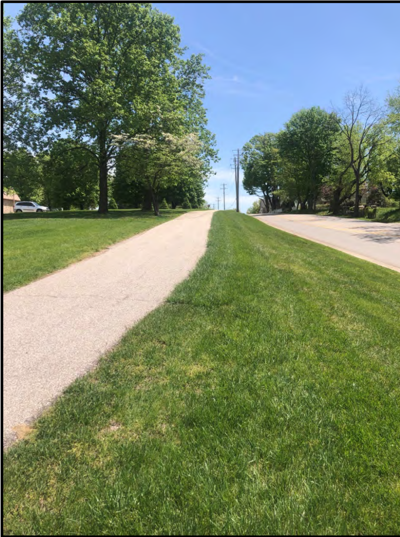
9. View east along SR 45. 5/4/2020
