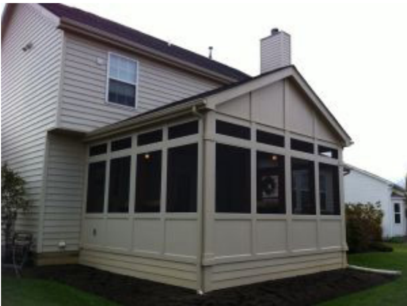
Sample screened porch
