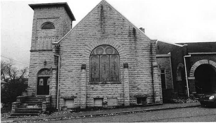
**Commented [HJ2]:** 8<sup>th</sup> Street view following replacement of broken window with glass block and 3 remaining windows replaced with glass block to match.
