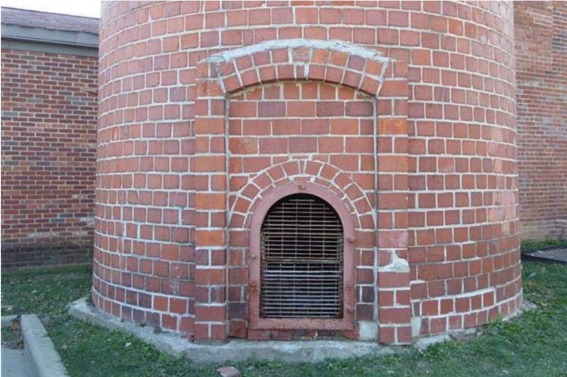
Photo 13 Opening at the base of the stack.
