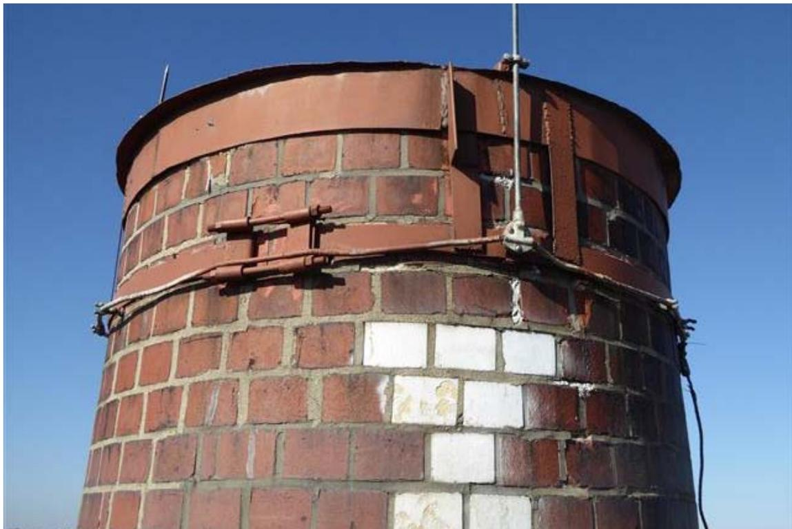
Photo 12 This prevents rain from falling inside but promotes freeze/thaw deterioration due to the “chimney effect” where warm, moist air rises and condenses on the inside face of the masonry.
