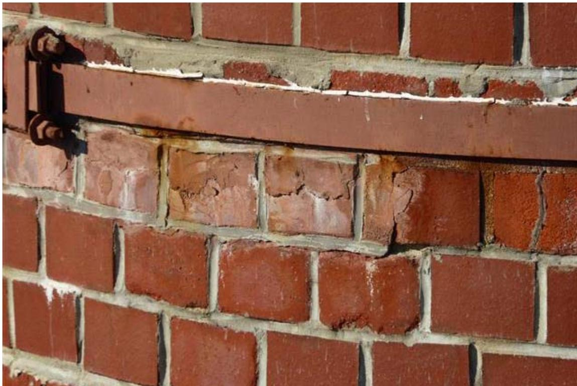
Photo 24 The patching material cracks and falls away itself.
